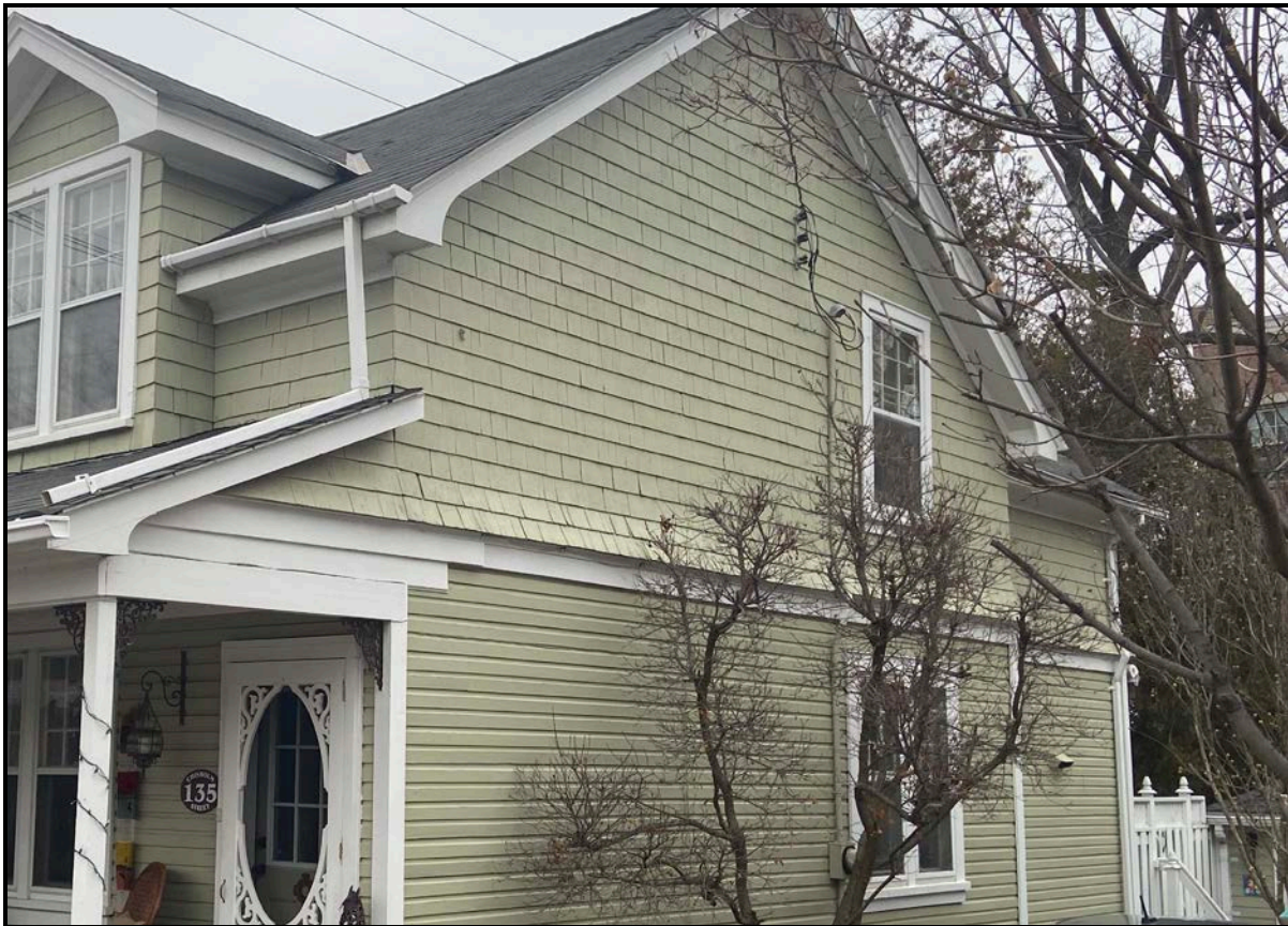
Siding on 135 Chisholm Street, showing the shingles and horizontal siding, 2024. Source: Town of Oakville Planning Staff
