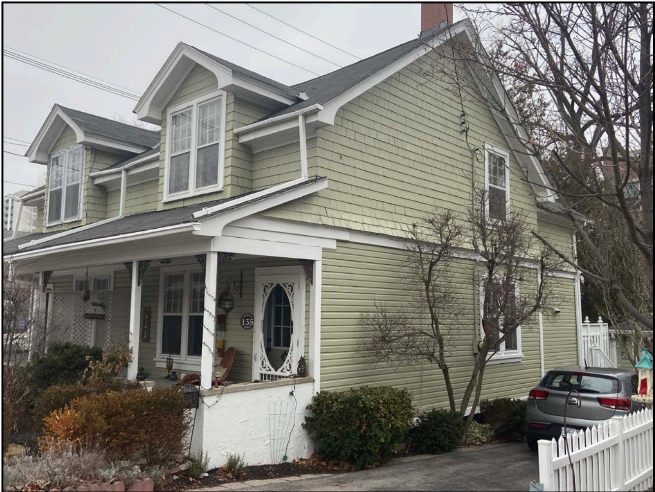
View of the west elevation (front) and south elevation of 135 Chisholm Street, 2024. Source: Town of Oakville Planning Staff
