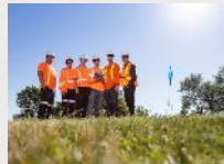
Utility locating / damage prevention
