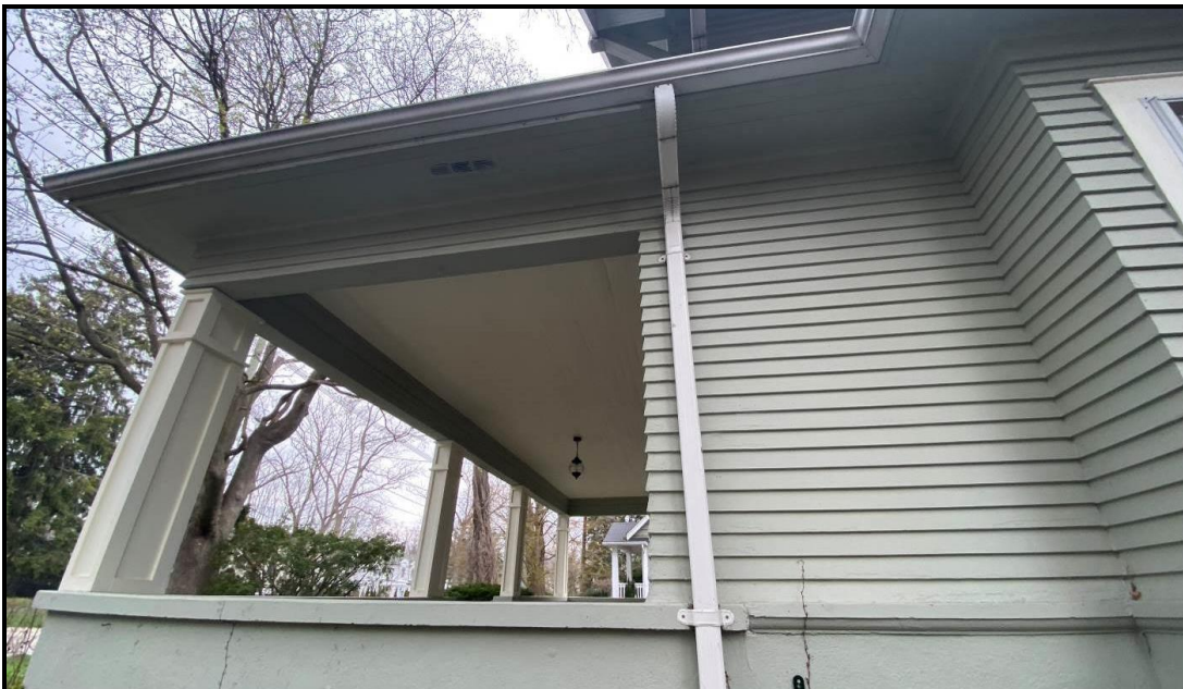
View of the front porch roof overhang with wooden soffit that goes around both sides of the house and acts as the roof on the projecting window on the west elevation, 2024. Source: Town of Oakville Planning Staff
