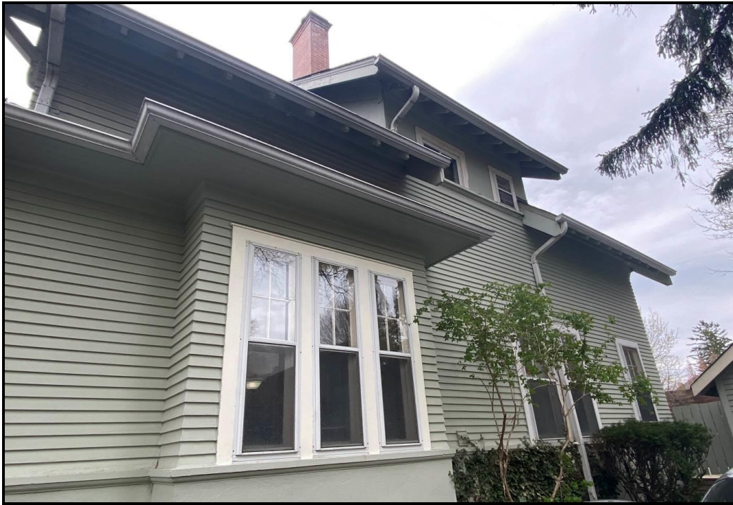
Shed dormer and unique porch roof overhang that wraps around both east and west elevations, with a projecting window, 2024. Source: Town of Oakville Planning Staff
