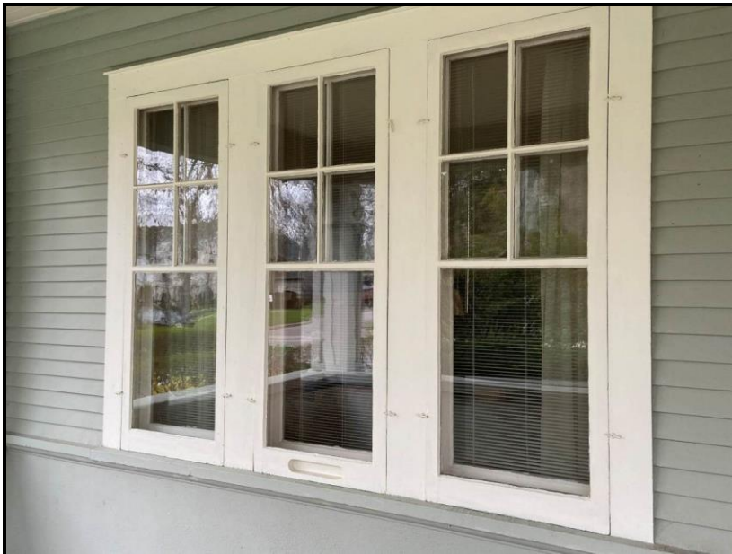
One set of the three windows on the first storey, showing the wooden trim and the historical multipaned windows and storm windows, 2024. Source: Town of Oakville Planning Staff
