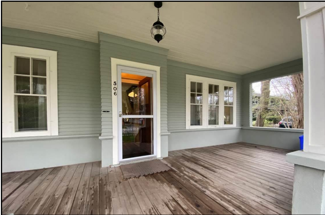
Front porch showing the wooden ceiling, flooring, the trim running along the foundation, and the projecting front door, 2024. Source: Town of Oakville Planning Staff
