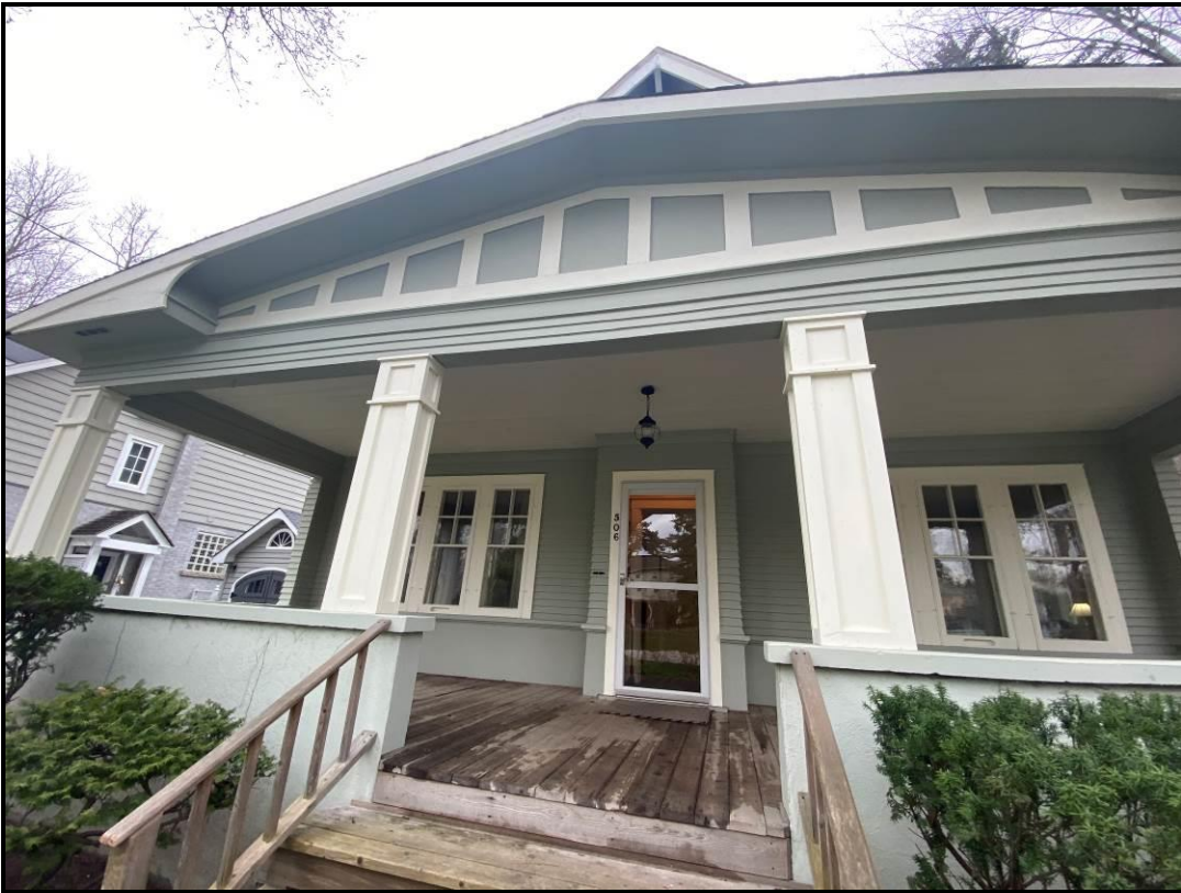
Wooden detailing on the porch showing the columns, half-timbering, the decorated edges, wooden trim detailing, and a concrete porch wall, 2024. Source: Town of Oakville Planning Staff
