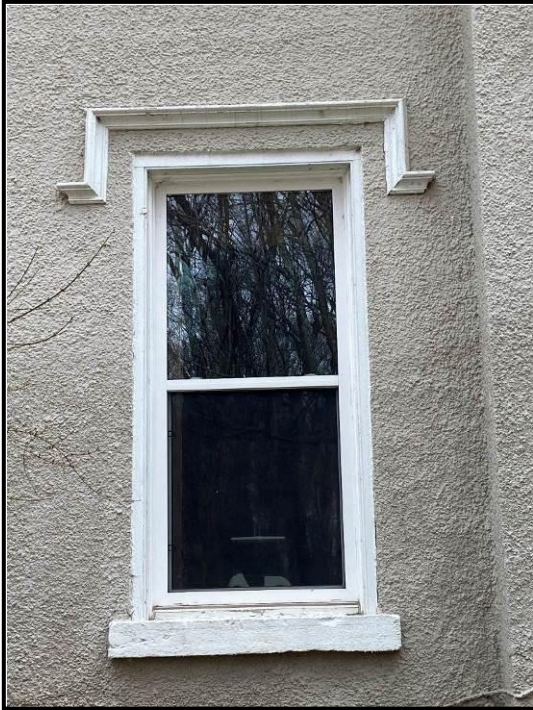
Close up of one of the windows with drip edge on the north elevation, 2024. Note the wood sills and frame. Source: Town of Oakville Planning Staff
