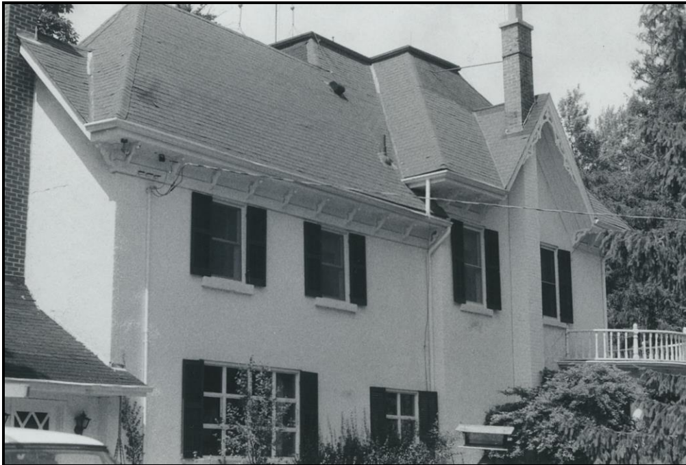
1977 photo showing the thick wooden muntins and square panes of glass on the first storey windows. Source: Town of Oakville planning files
