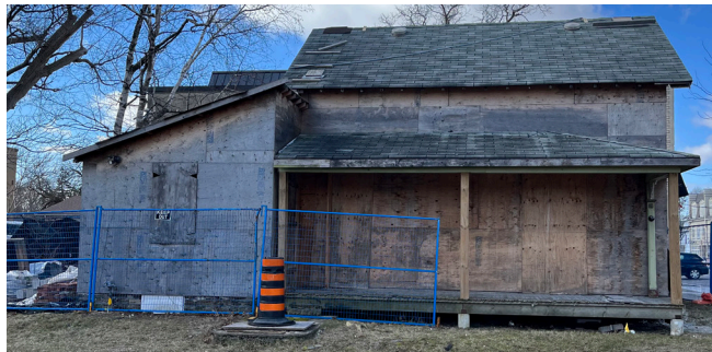
East elevation of 42 Lakeshore Road West (ERA, 2023).
