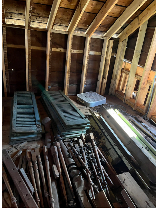
Salvaged items on second floor (ERA, 2023).
