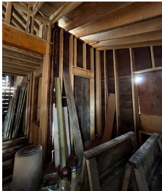
Structural reinforcement on first floor (ERA, 2023).
