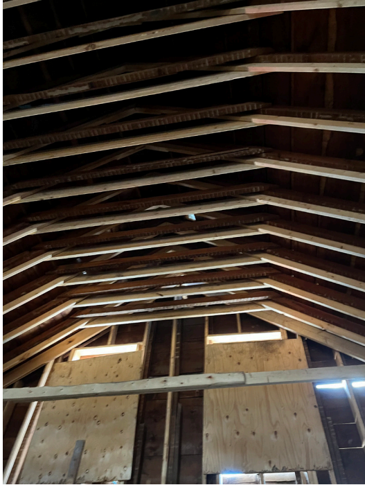
Structural reinforcement along roofline (ERA, 2023).
