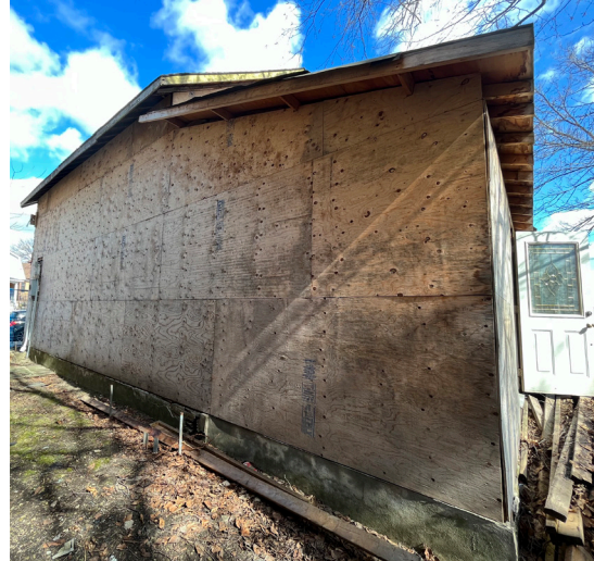
West elevation of 42 Lakeshore Road West (ERA, 2023).
