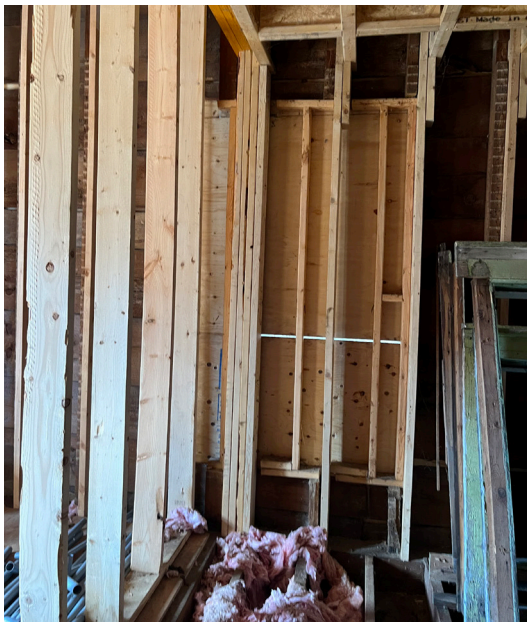
Structural reinforcement on first floor (ERA, 2023).
