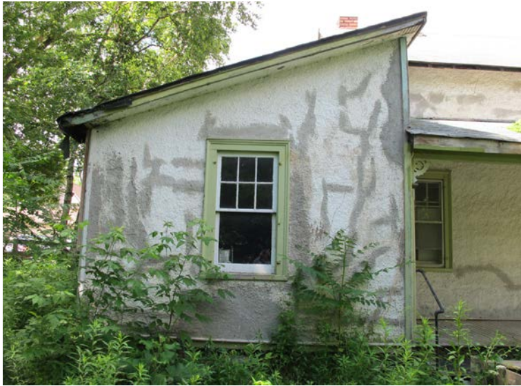
Rear portion of east elevation (ERA, 2011).
