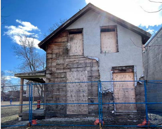
Principal (north) elevation of 42 Lakeshore Road West (ERA, 2023).
