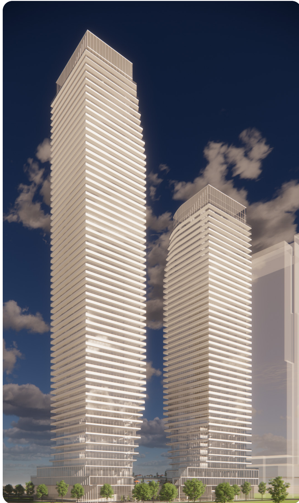
Tower Southeast Street View
