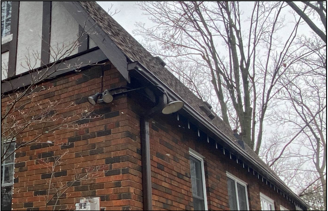
The house contains many of its original wood windows. Typical of the Tudor Style, there is a variety of styles and sizes of windows throughout the house. On the south and north elevations, the original 6/1 wood sash windows and 6-pane wood fixed windows remain, along with their wood storms.
