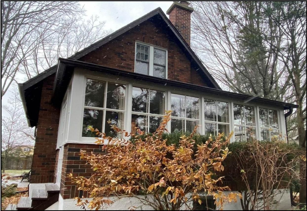
West elevation of the house, showing the enclosed side porch that now faces the street. Source: Town of Oakville Planning Services Staff
