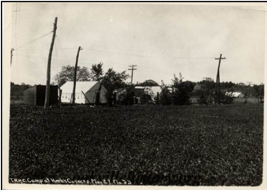
Another photo showing a highway construction camp at Heek’s Corners, circa 1915. It is not clear which direction this photo faces Source: Oakville Historical Society
