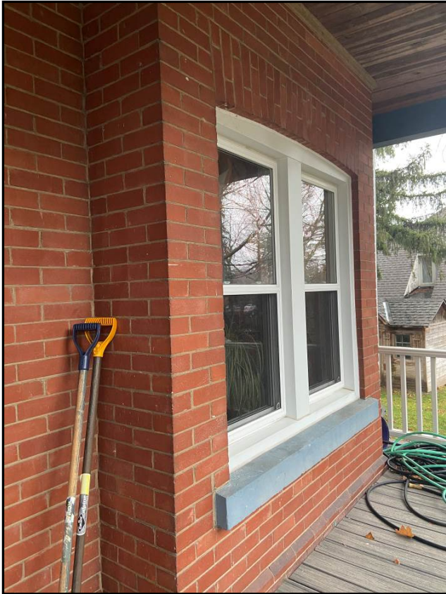
Photo showing the brick projections for the on the front porch and wooden ceiling.
