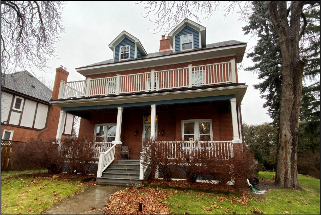
Front elevation of the house, 2024. Town of Oakville Planning/Heritage Planning
