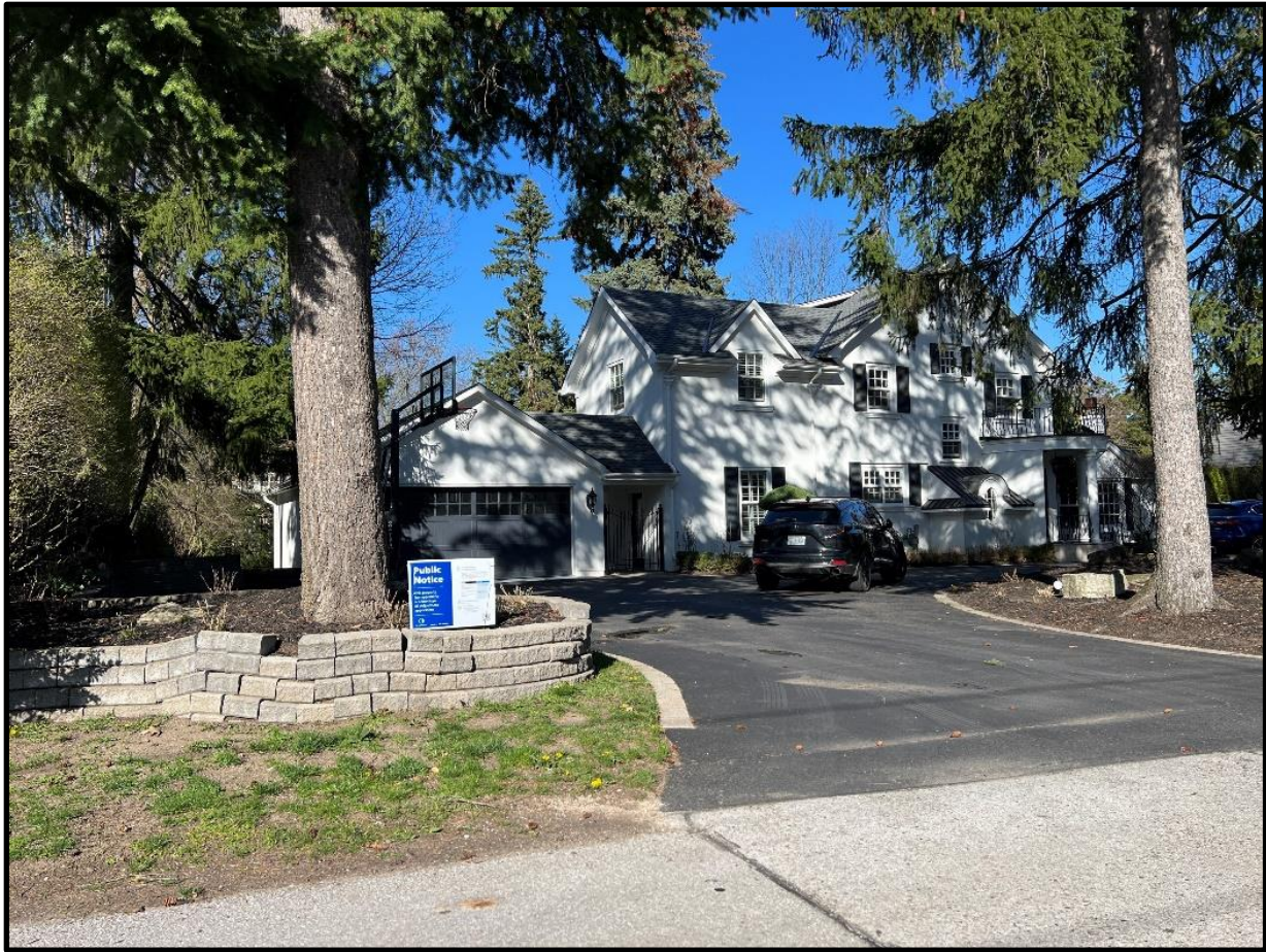
317 Gloucester Avenue – Existing Dwelling
