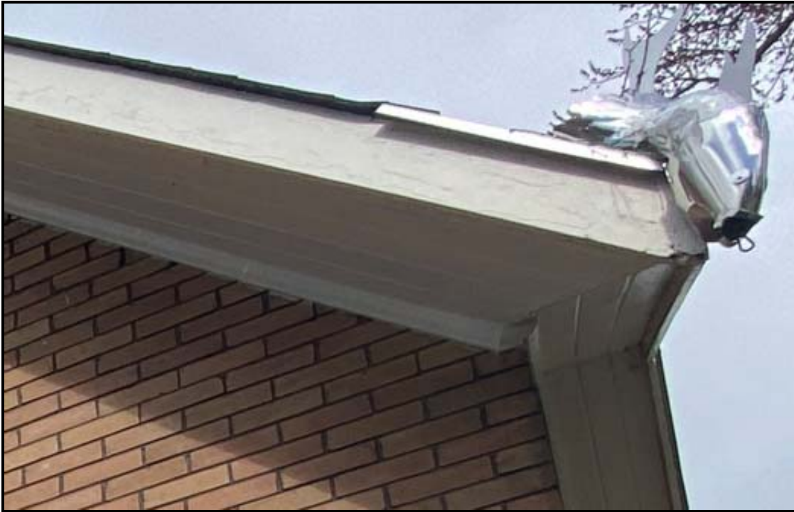
Close-up of offset gable on the front façade and the house's wooden soffits and fascia. A rain chain has been installed on this unique corner to divert rainwater from the roof. Source: Town of Oakville Planning Staff
