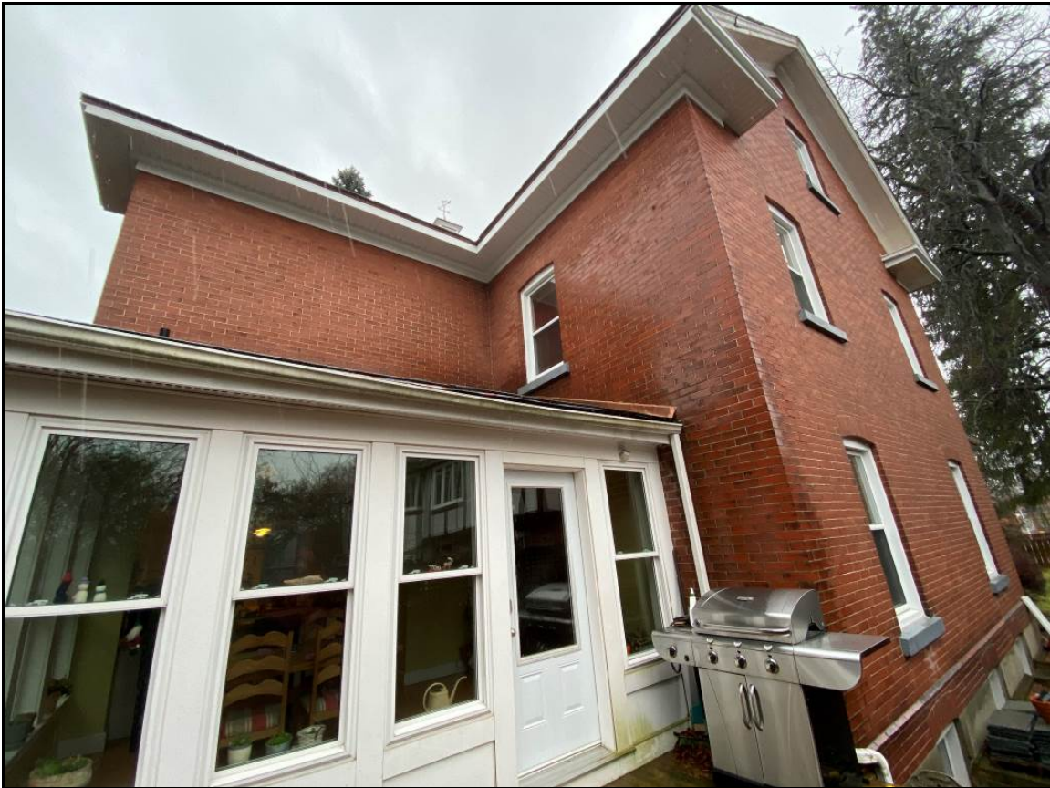
East (rear) and north elevation showing the covered sunroom and rear wing on the left.
