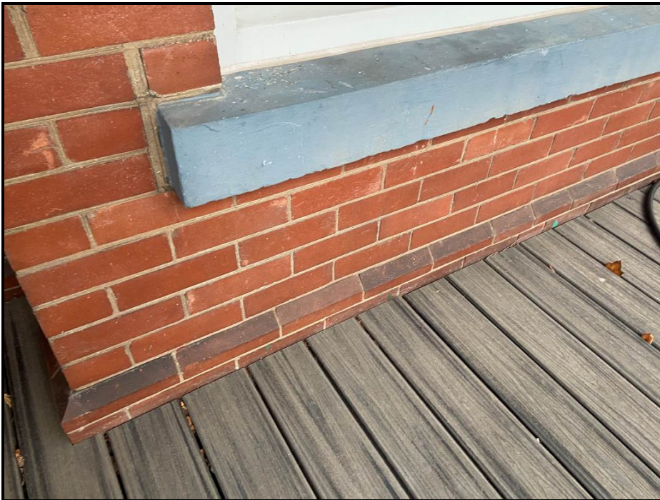
Brick footing running along the porch and house.
