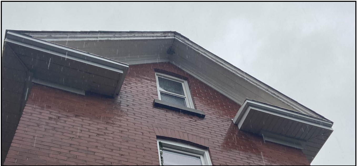
Cornice returns on the gabled sides and frieze.
