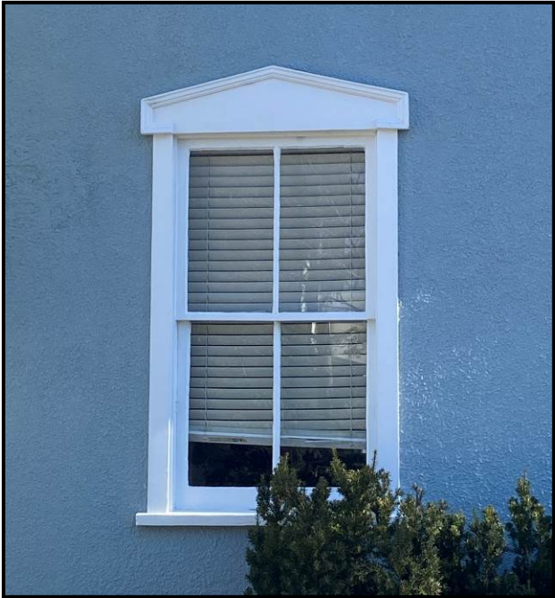
Left: Close up of one of the windows. This one does not have its storm window, but we can see the wooden sash, the pediment, and wooden frame. Source: Planning Services staff photo, 2024.
