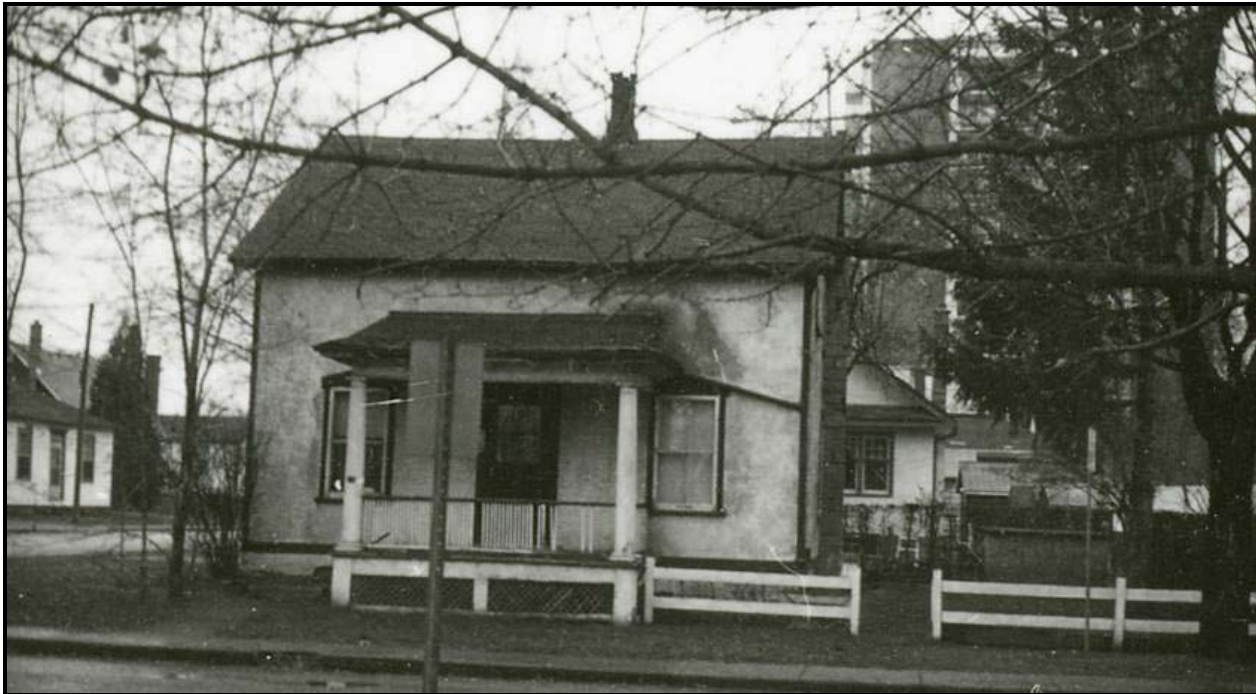
1971 photo showing the historic Neoclassical porch on the front façade. A central chimney was also present on the roof and was likely removed later. Note the wooden trim on each corner of the house and along the foundation that is still present. Source: Canadian Inventory of Historic Buildings, Parks Canada.
