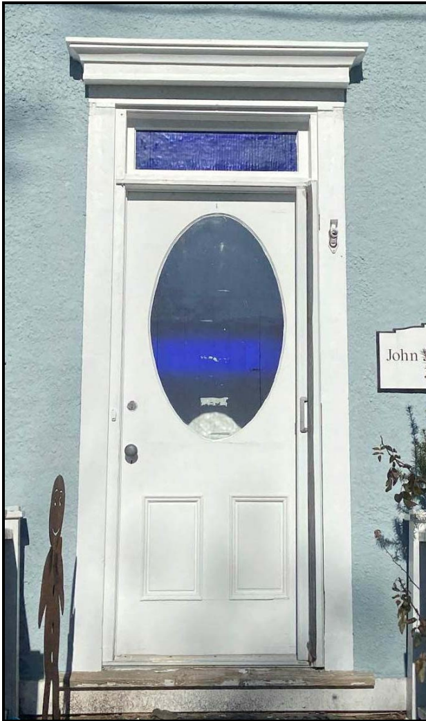
Left: The front door the entablature and transom window.
