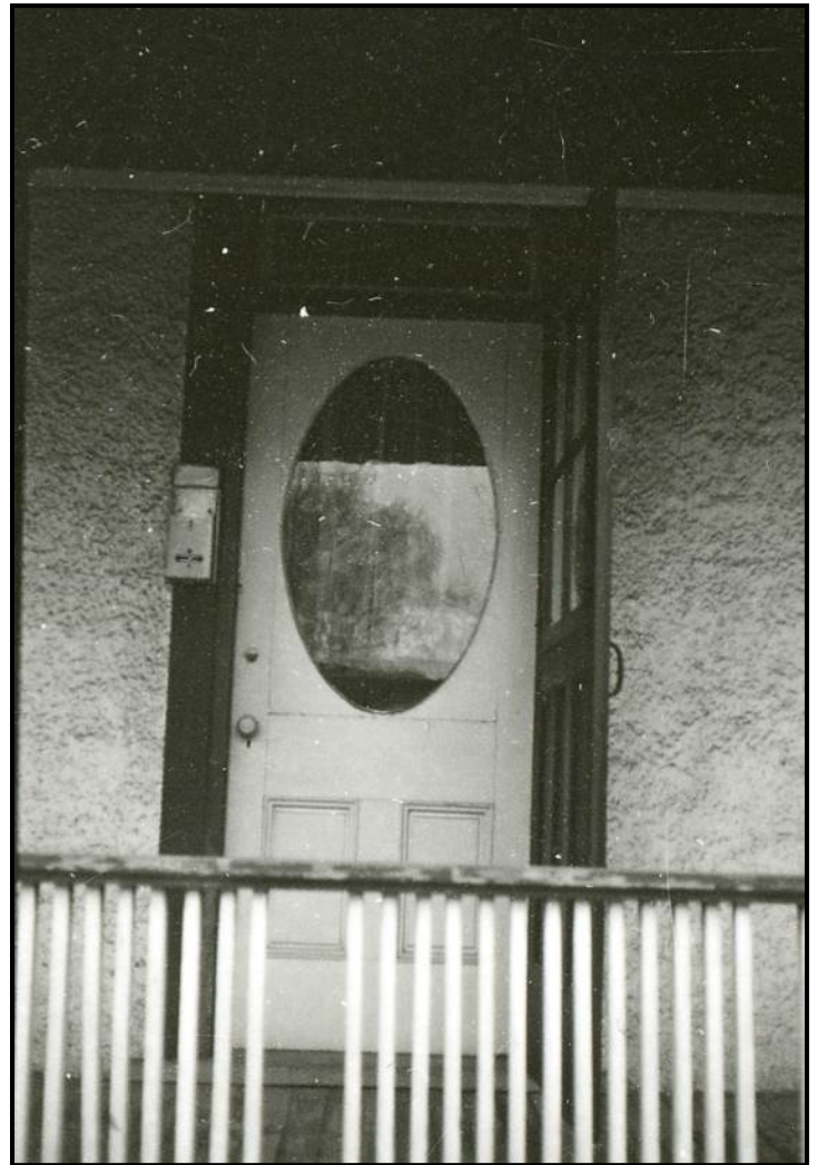
Right: The door in 1971. Note the porch roof was where the entablature now sits, which was probably added when the porch was removed post-1971. Source: Canadian Inventory of Historic Buildings, Parks Canada.
