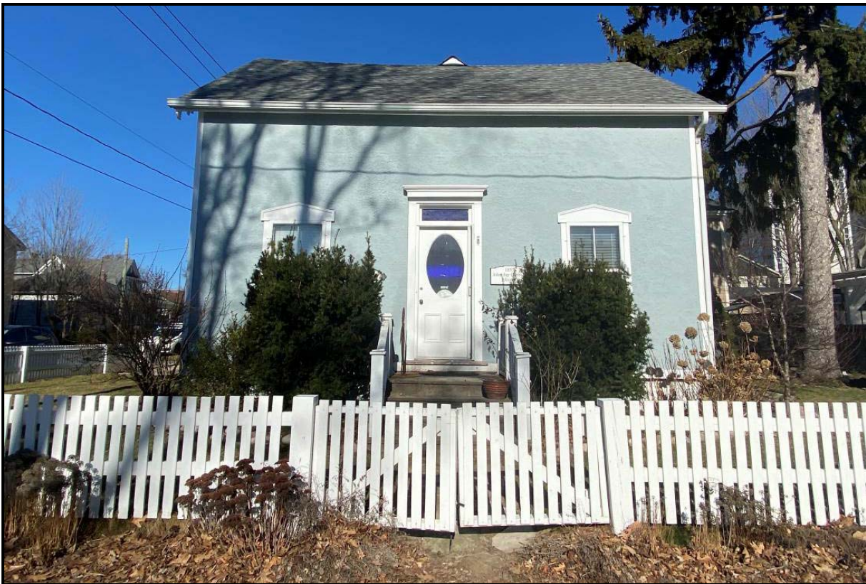
South elevation with the front door. Source: Planning Services staff photo, 2024.
