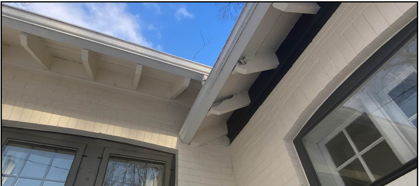
Wooden soffit and exposed eaves on the front façade. Source: Town of Oakville Planning Services Staff
