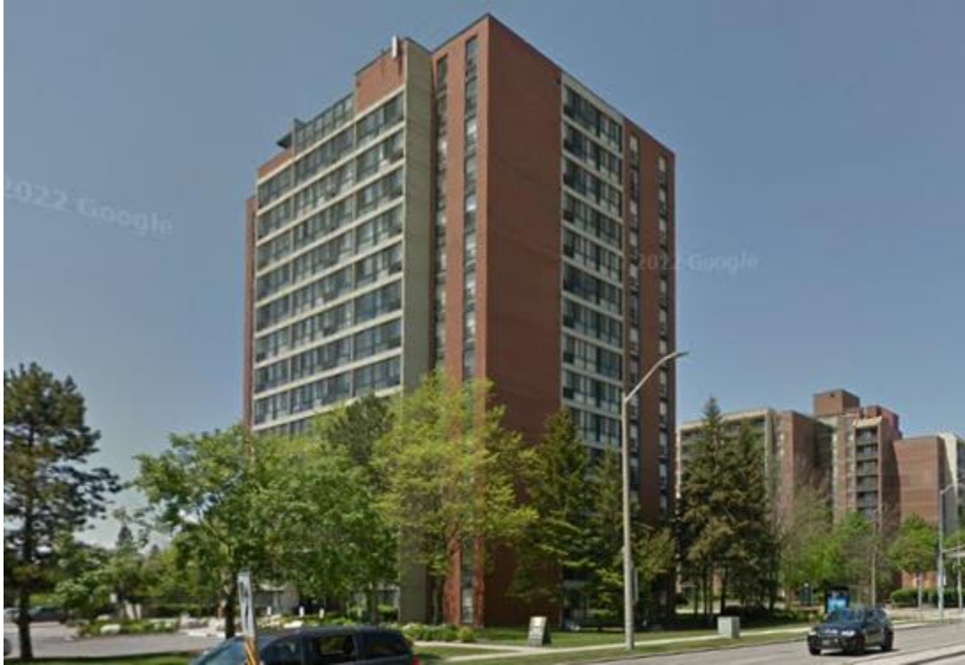
Surrogate site #2, residential condo building (6550 Glen Erin Dr, Mississauga)
