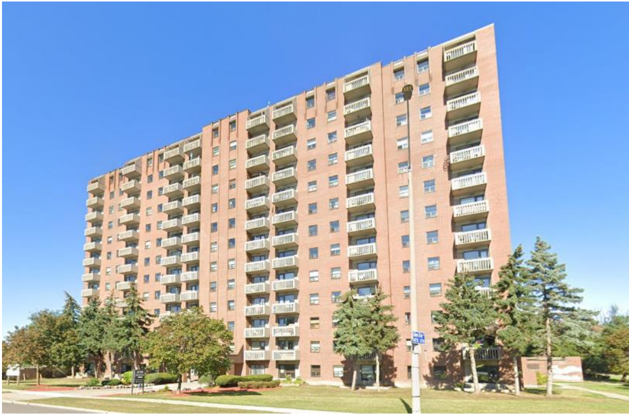
Surrogate site #3, residential condo building (6719 Glen Erin Dr, Mississauga)
