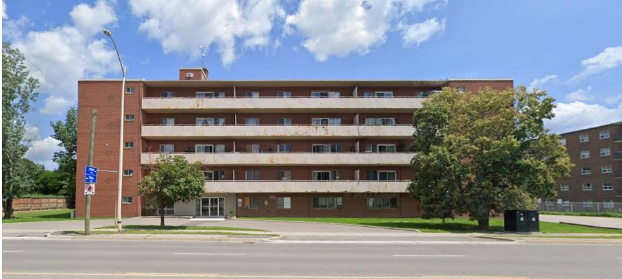
Surrogate site #4, residential condo building (263 Ontario St N, Milton)
