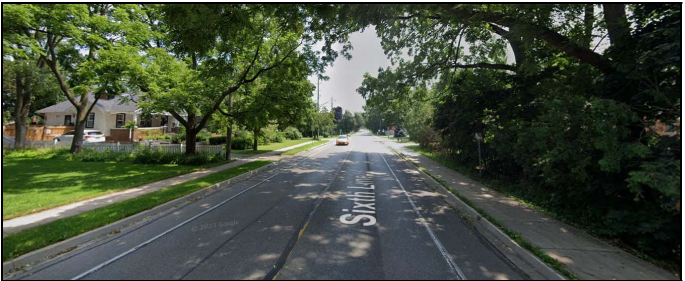
Looking south on Sixth Line with the subject property on the left, 2023. Source: Town of Oakville Planning Services Staff
