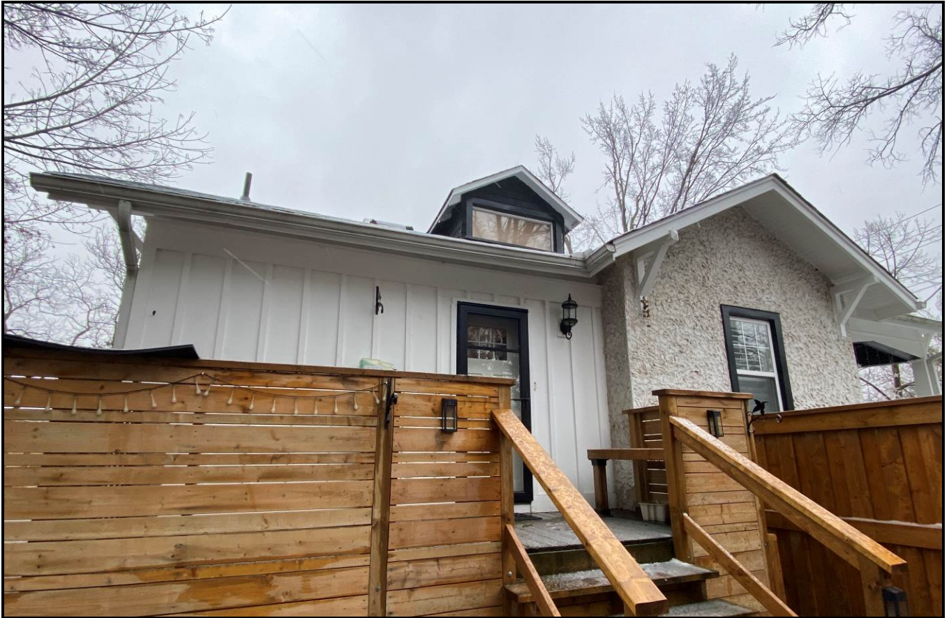
West elevation close up with the small side gabled dormer and enclosed porch. Town of Oakville Planning Services Staff
