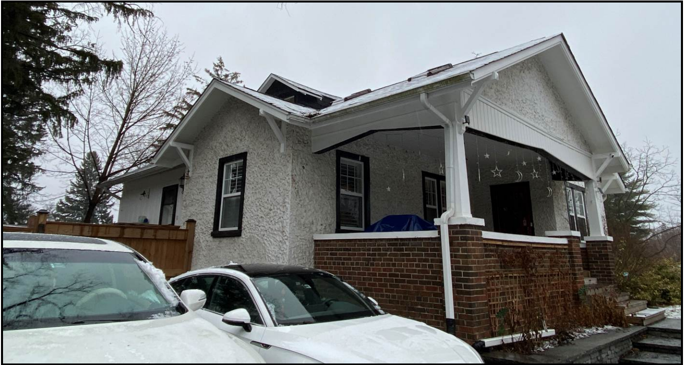
East and north elevations of the house, showing the enclosed porch-turned-living space on the far left. Source: Town of Oakville Planning Services Staff
