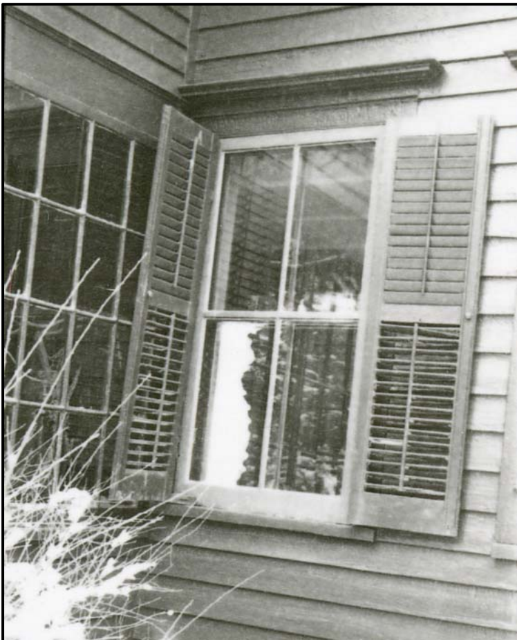
Multi-paned wood windows on the c.1830s house and front portico wing. January 2024. Source: Town of Oakville Planning Services staff
