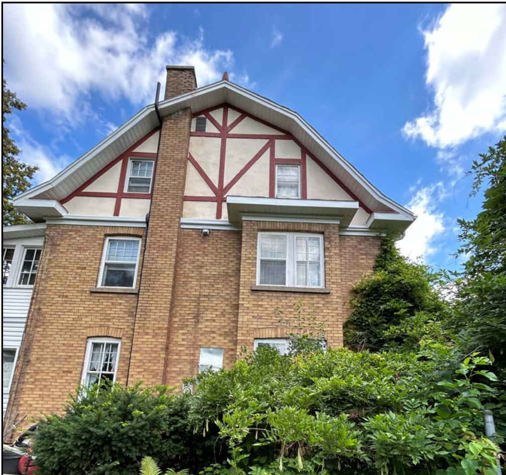
View of west elevation showing the half timbering and stucco with buff brick cladding. Source: Town of Oakville Planning Services Staff
