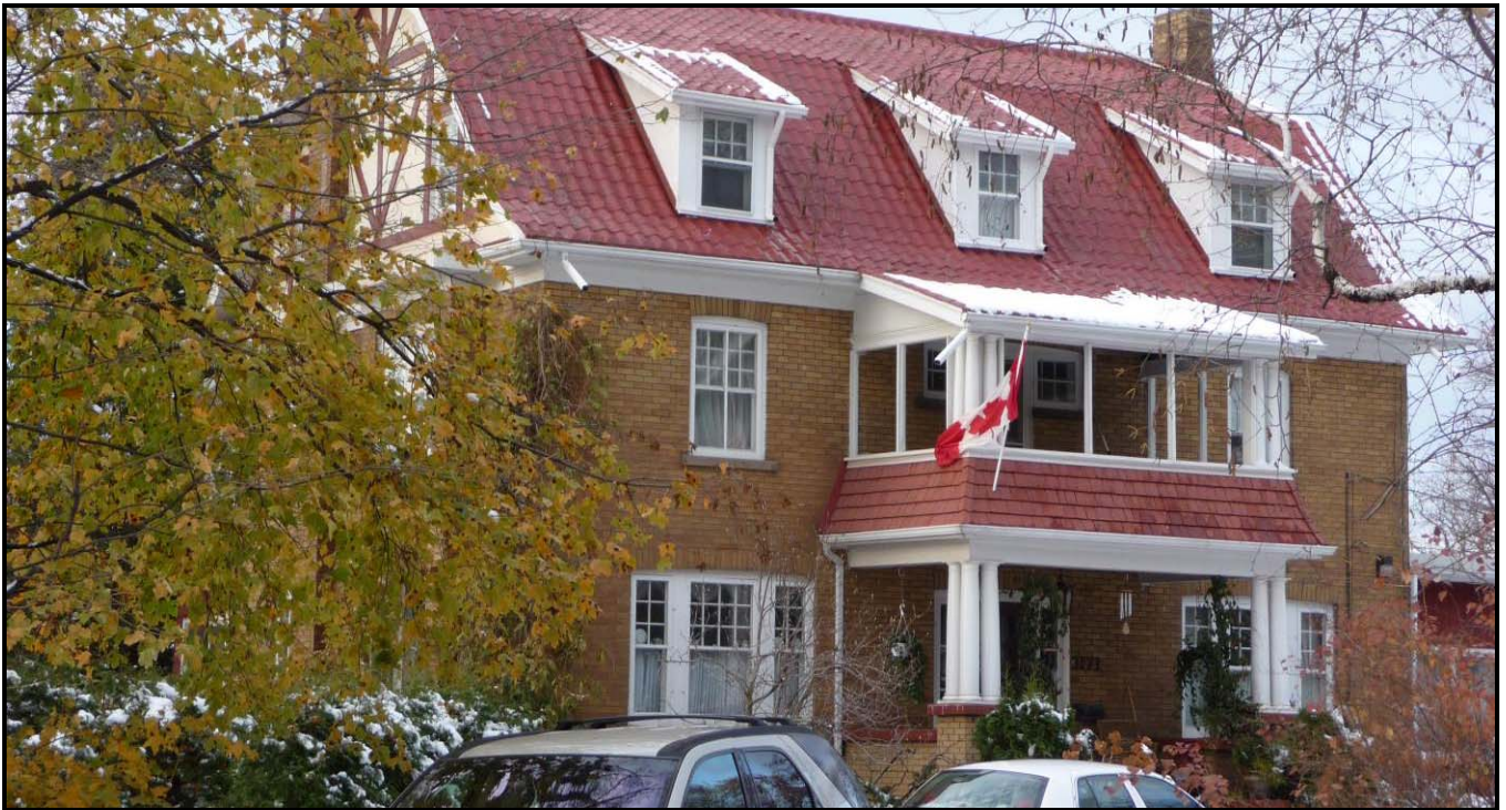
Photo of the south elevation, more clearly showing buff brick cladding, covered porch with second storey, and red metal roof with dormers, 2008. Source: Town of Oakville/Oakville Heritage Planning
