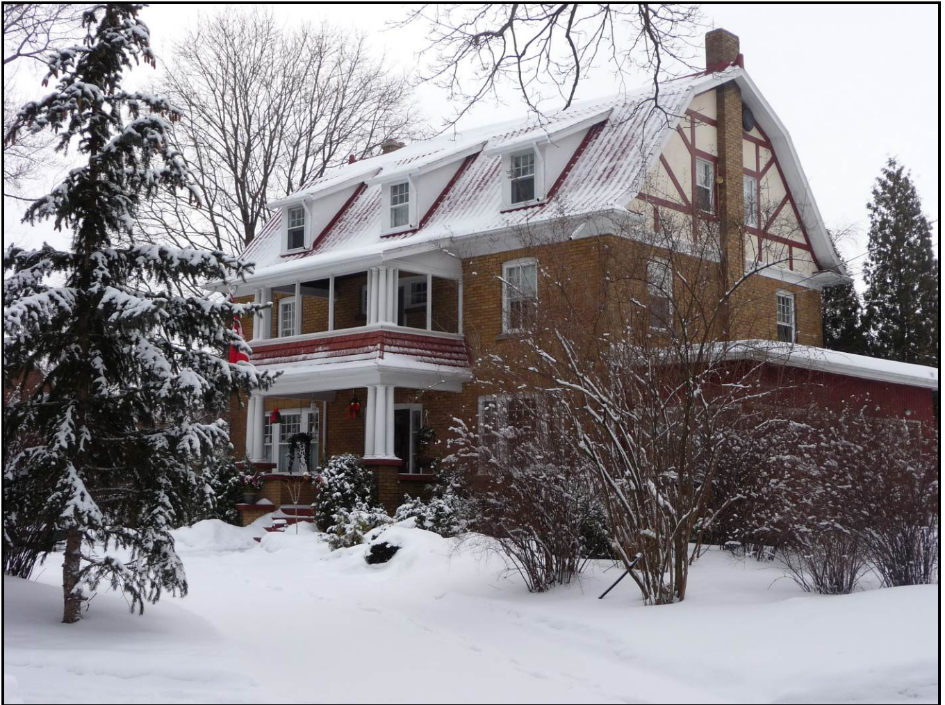
View of the home from the street, depicting some of its heritage elements such as the gambrel roof, dormers, and half-timbering design, 2008. Source: Town of Oakville Planning Services Staff
