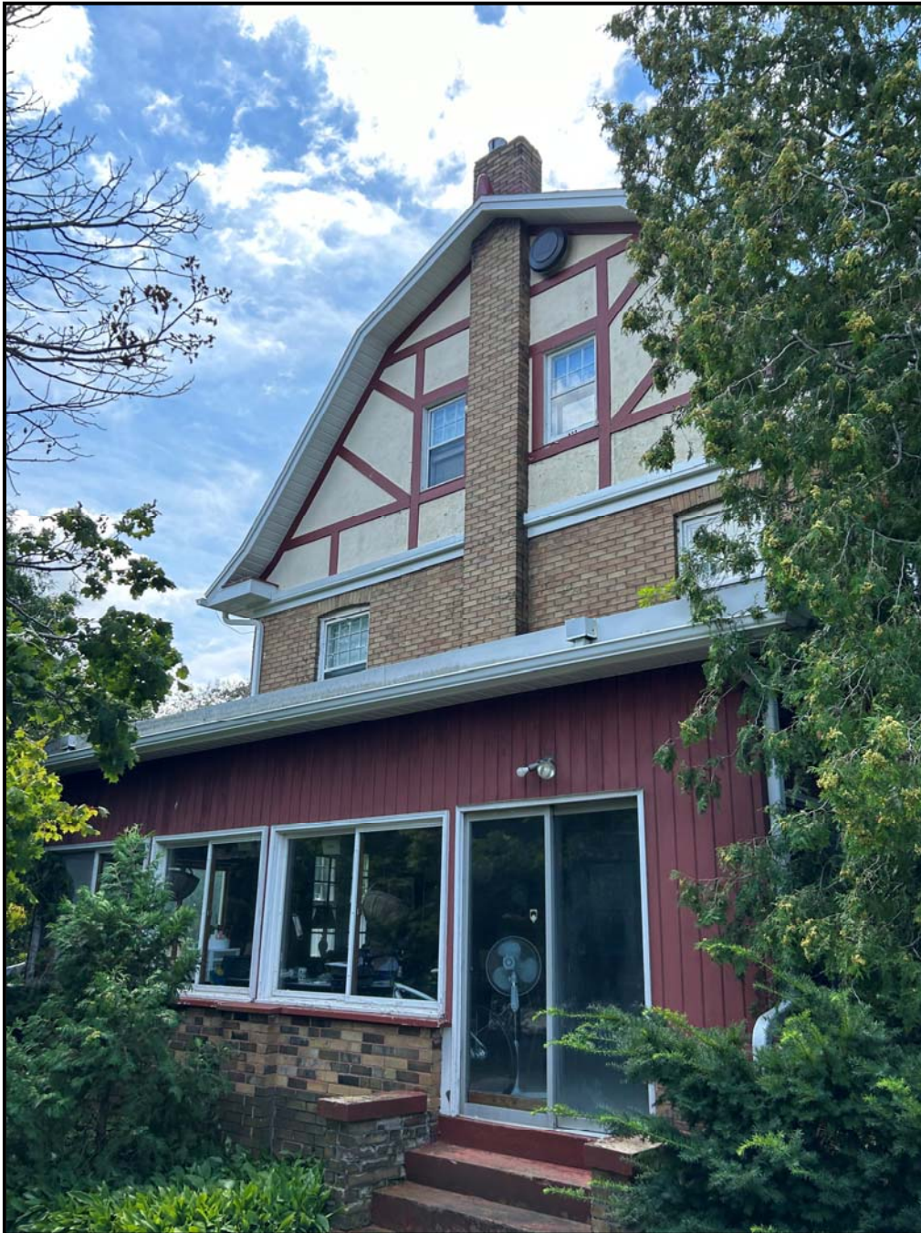
View of the east elevation with covered sun porch. It appears to also have brick cladding with brick piers on the steps. Source: Town of Oakville Planning Services Staff
