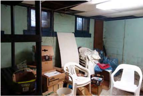
3171 LAKESHORE ROAD W: Basement – unfinished - concrete block foundation
