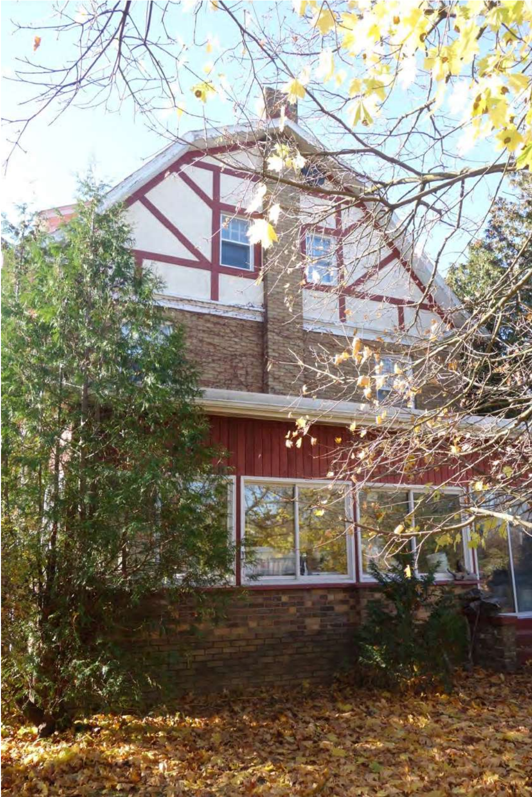
3171 LAKESHORE ROAD W: East side elevation – 1-storey porch has been enclosed
