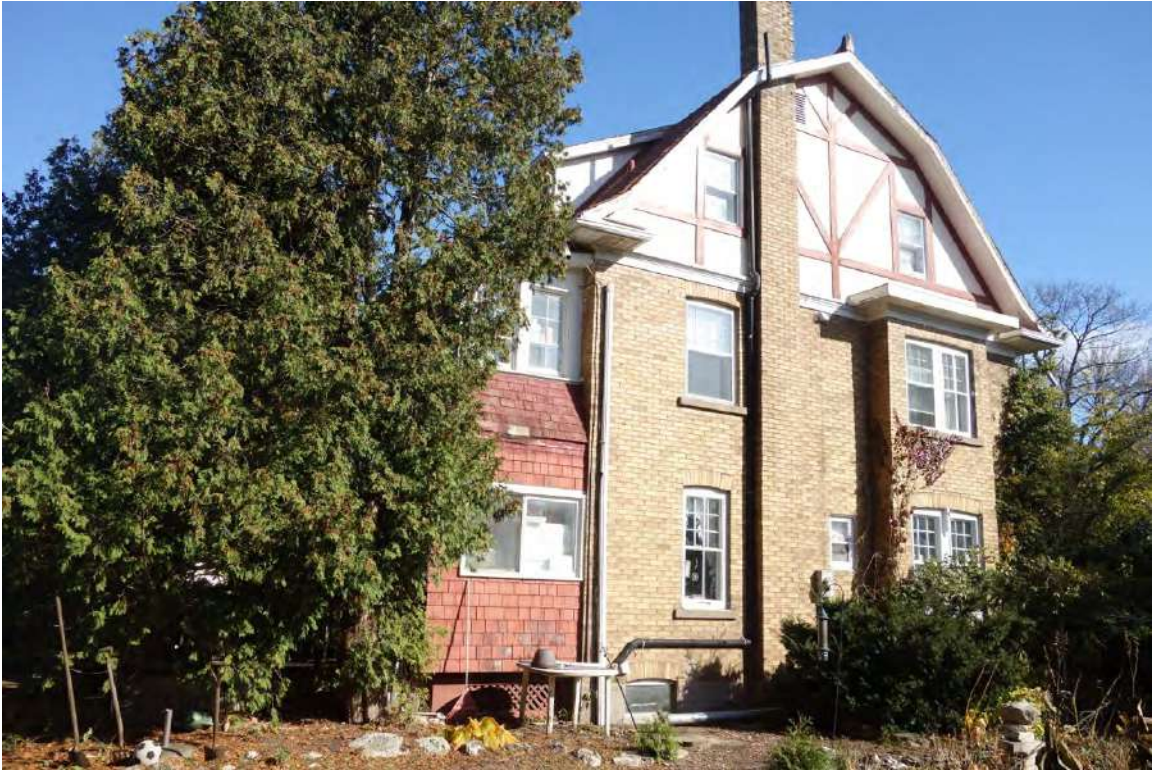
3171 LAKESHORE ROAD W: West side elevation
