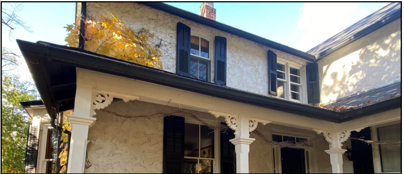
Projecting eaves above the porch. Source: Town of Oakville Planning Services Staff
