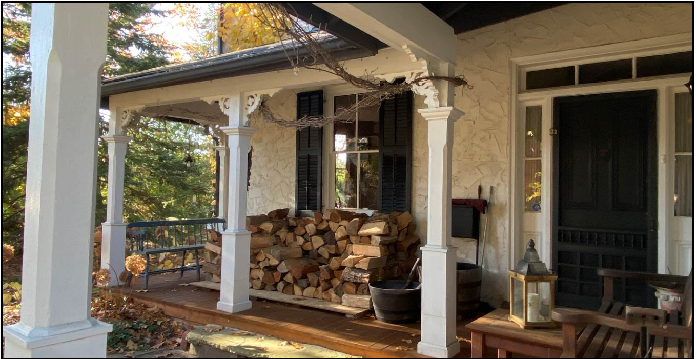
Verandah on the south elevation looking northwest. Historically, a path through the gate on the west elevation would have led here. Source: Town of Oakville Planning Services Staff
