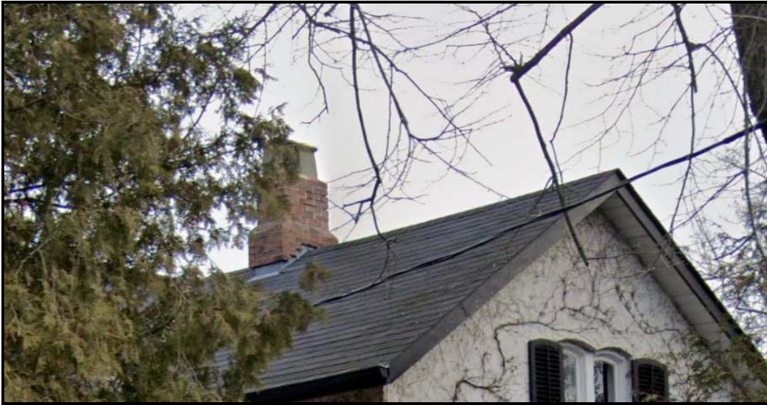
Current chimney. Source: Google Street View
