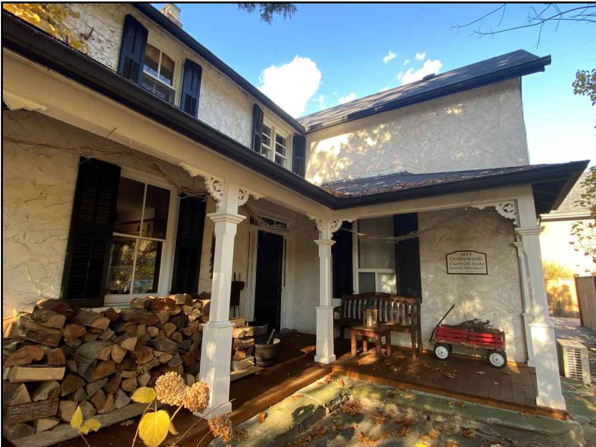
Verandah on south elevation, looking northeast. Source: Town of Oakville Planning Services Staff
