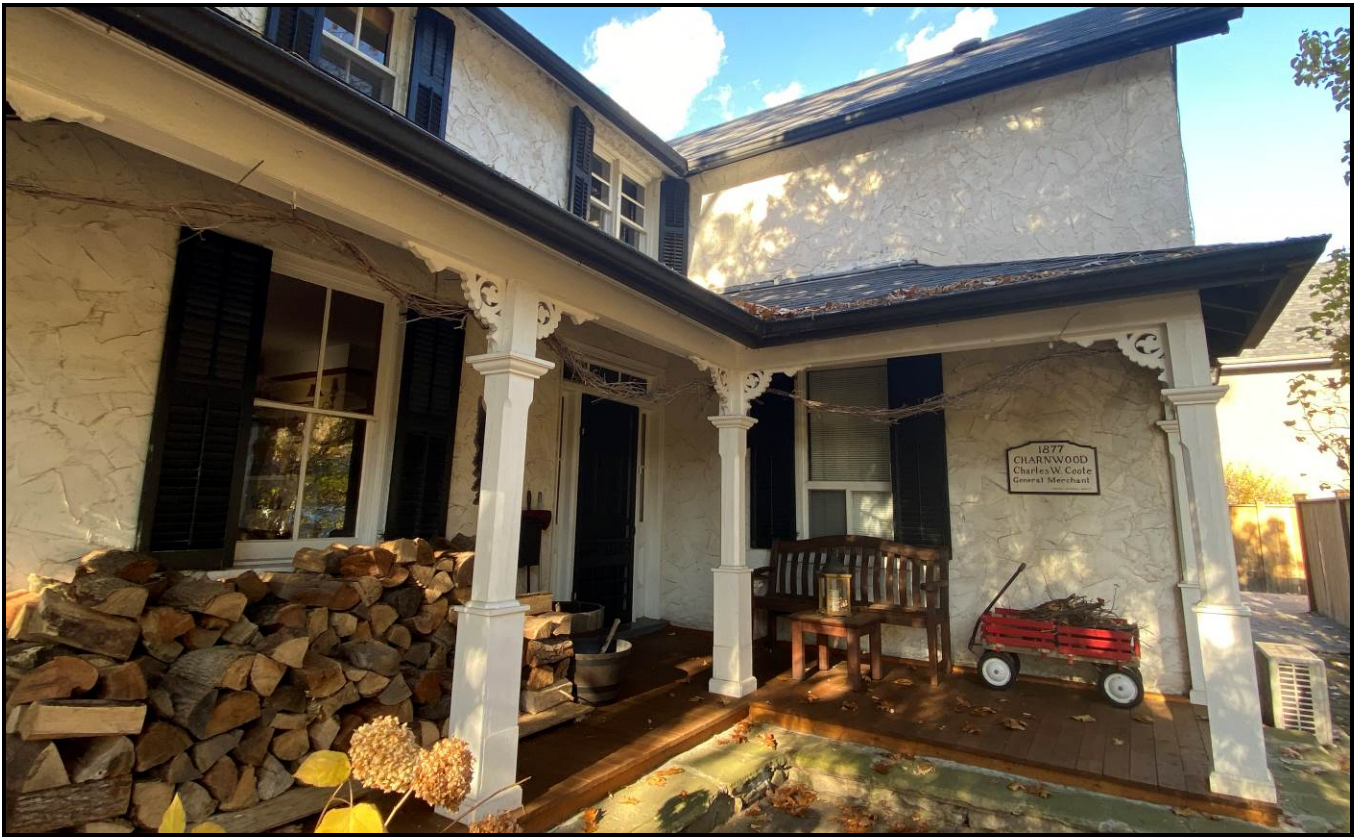
South elevation. Source: Town of Oakville Planning Services Staff
