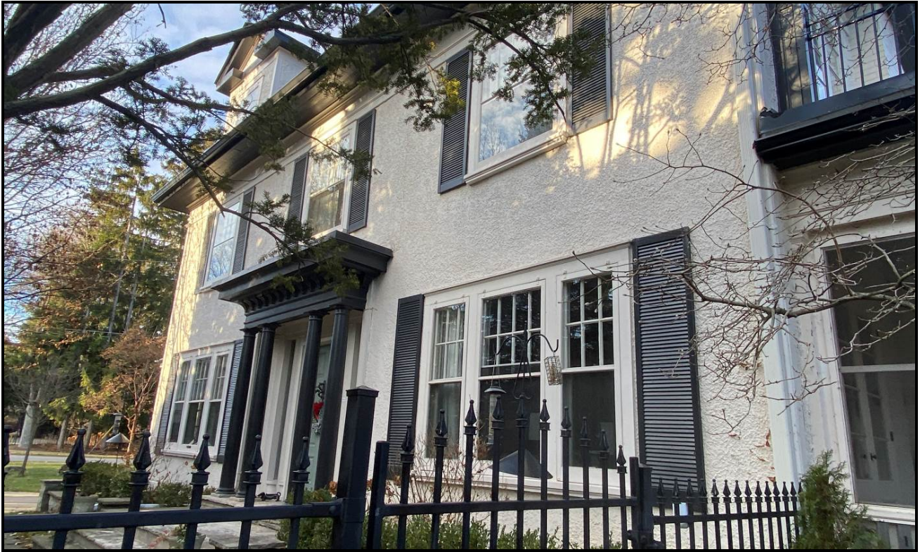
South elevation, 2023. Source: Town of Oakville Planning Services Staff
