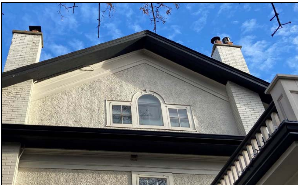
Palladian window on the west elevation. A matching one is on the east elevation. Source: Town of Oakville Planning Services Staff
