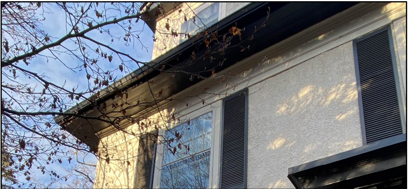
Close-up of the friezeboard and wooden soffit. Source: Town of Oakville Planning Services Staff
