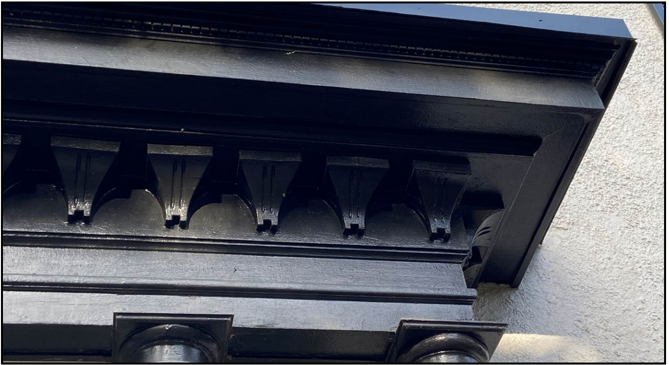
Close-up of the wooden detailing on the portico. Note the intricate dentil detailing. Source: Town of Oakville Planning Services Staff
