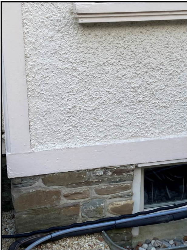
Left: close up of stucco siding and timber edging. Right: One of the chimneys on the west elevation. Source: Town of Oakville Planning Services Staff
