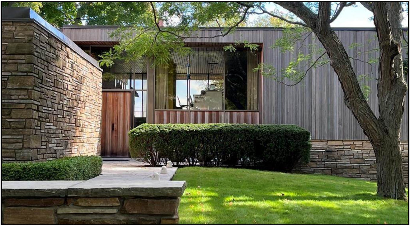
North elevation (front façade) of the house, showing the door half-hidden behind the garage structure, and the different cladding materials. Source: Phinney Real Estate/Oakville, Milton and District Real Estate Board
