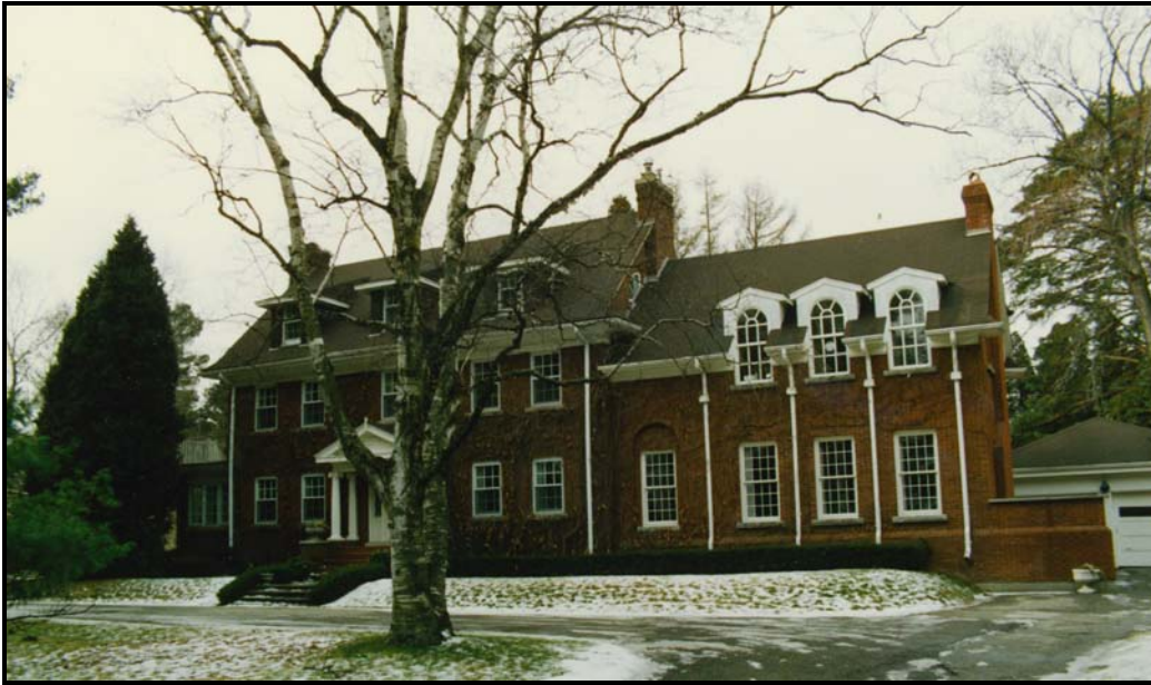
Circa 1990s historical photo of the house, showing the two chimney locations of the original portion of the house. Source: Town of Oakville files.
