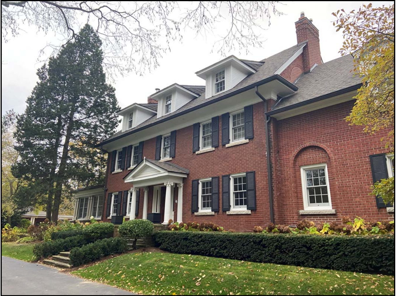
South elevation of the property, 2023. Source: Town of Oakville Planning Services Staff
