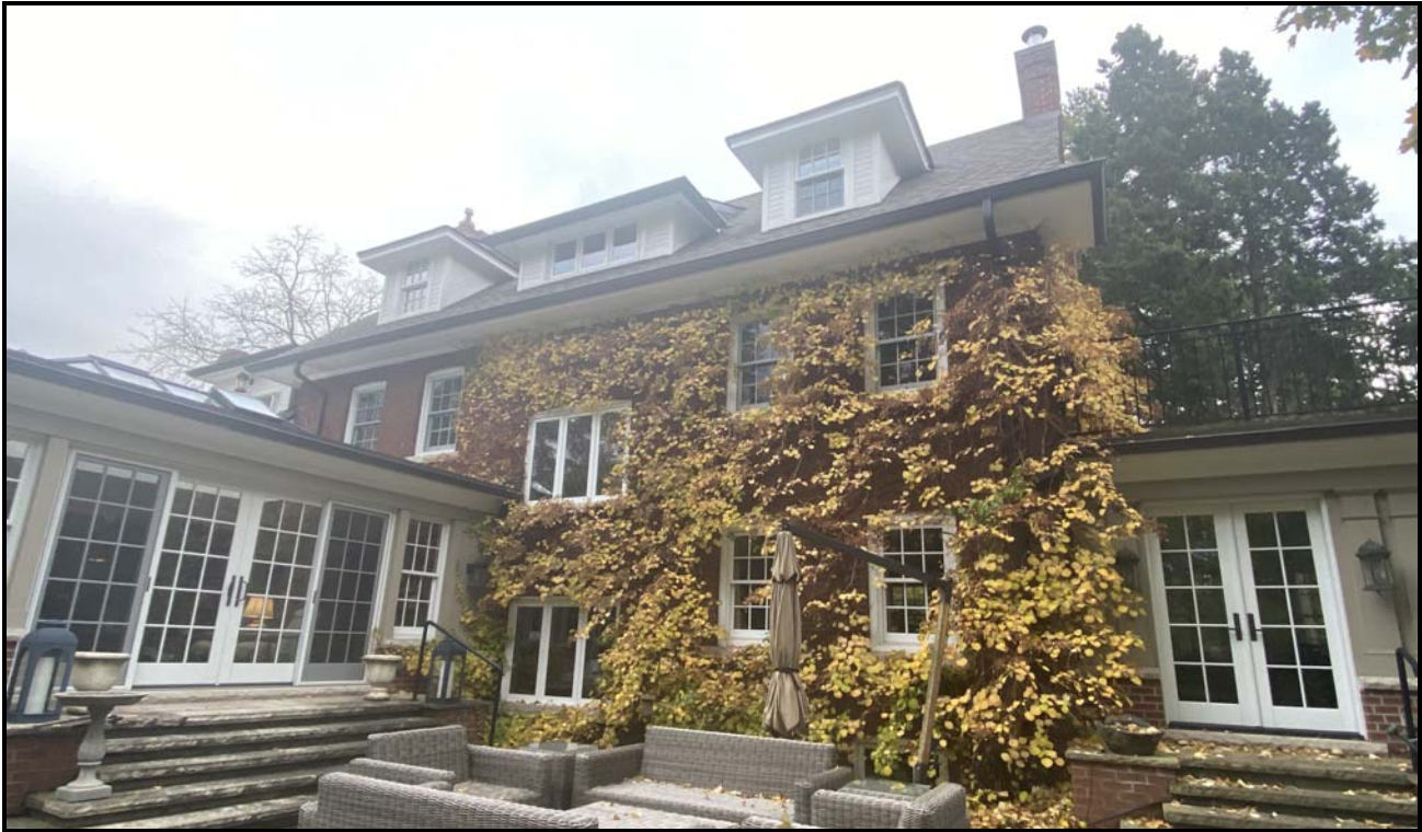
North elevation looking south. Source: Town of Oakville Planning Services Staff
