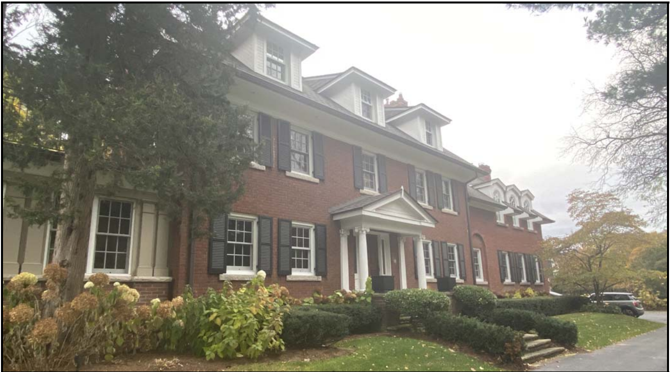
South elevation looking northeast. Source: Town of Oakville Planning Services Staff
