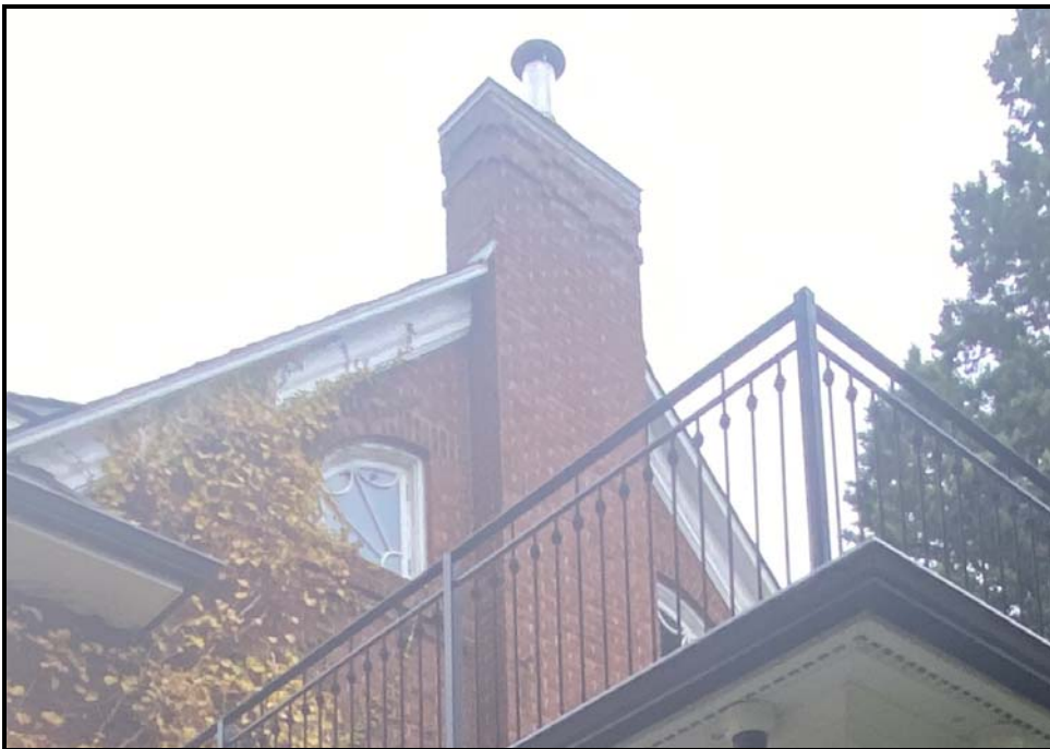
Chimney close-up showing the dentil detailing.
