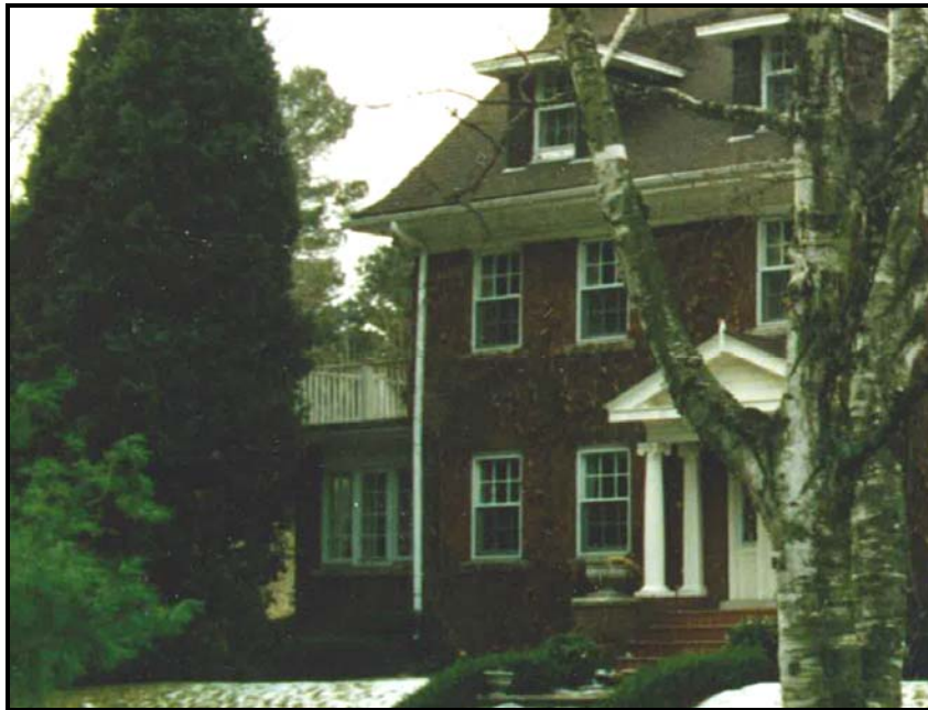
View of the former enclosed sunporch that was likely original to the house. Source: Town of Oakville Planning files
