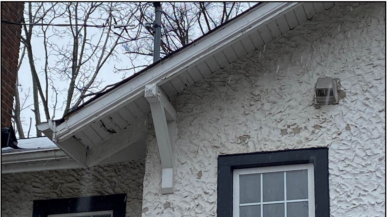
Close up of one of the wooden brackets that are spaced underneath the eaves, as well as wooden soffit and fascia. Source: Town of Oakville Planning Services Staff
