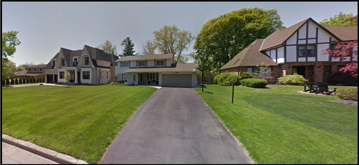
1594 Venetia Drive – Existing Dwelling
