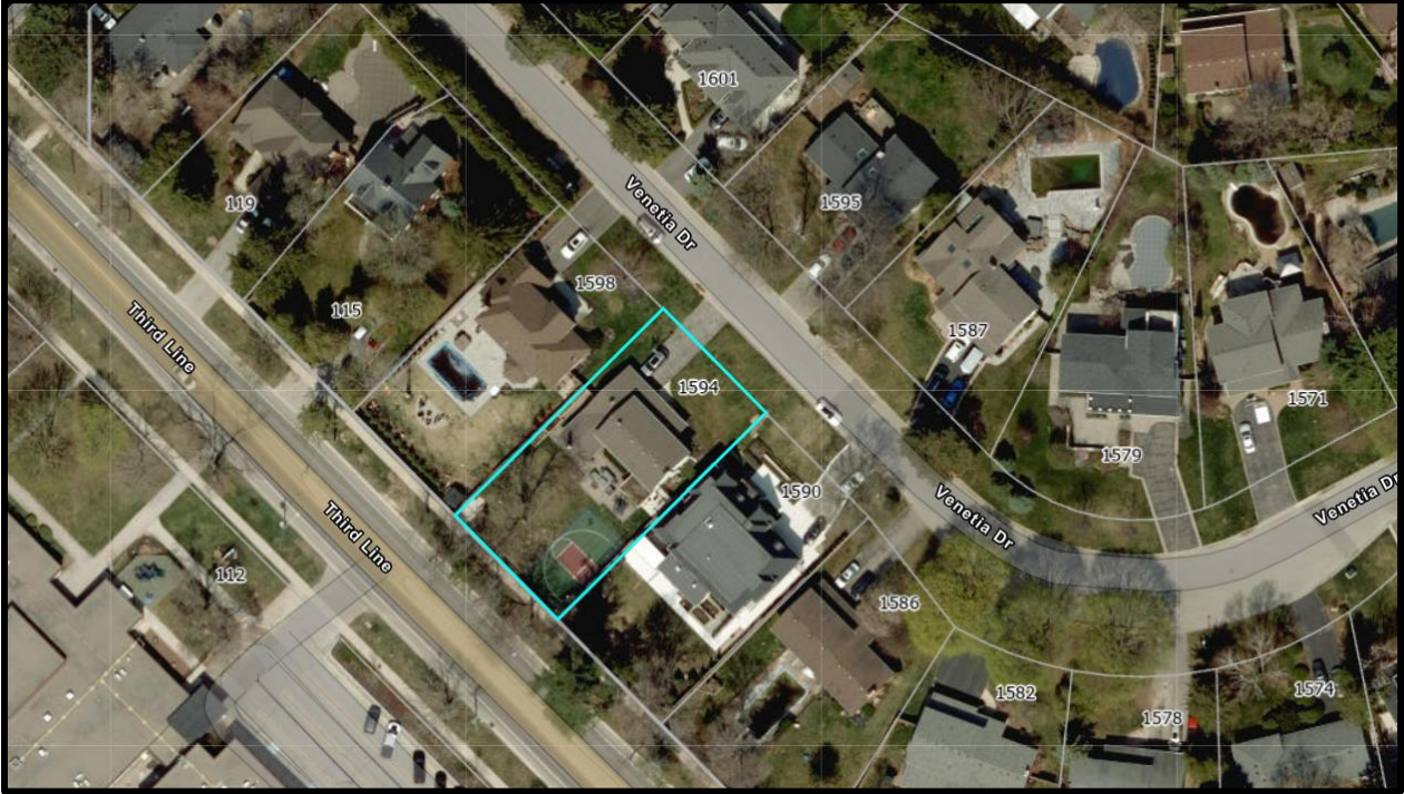
Aerial photo of 1594 Venetia Drive
