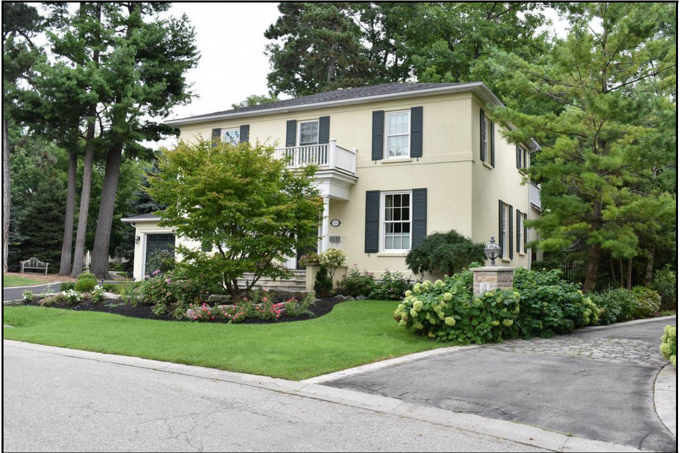
West elevation of the subject property, 2018. Source: Town of Oakville Planning Services Staff
