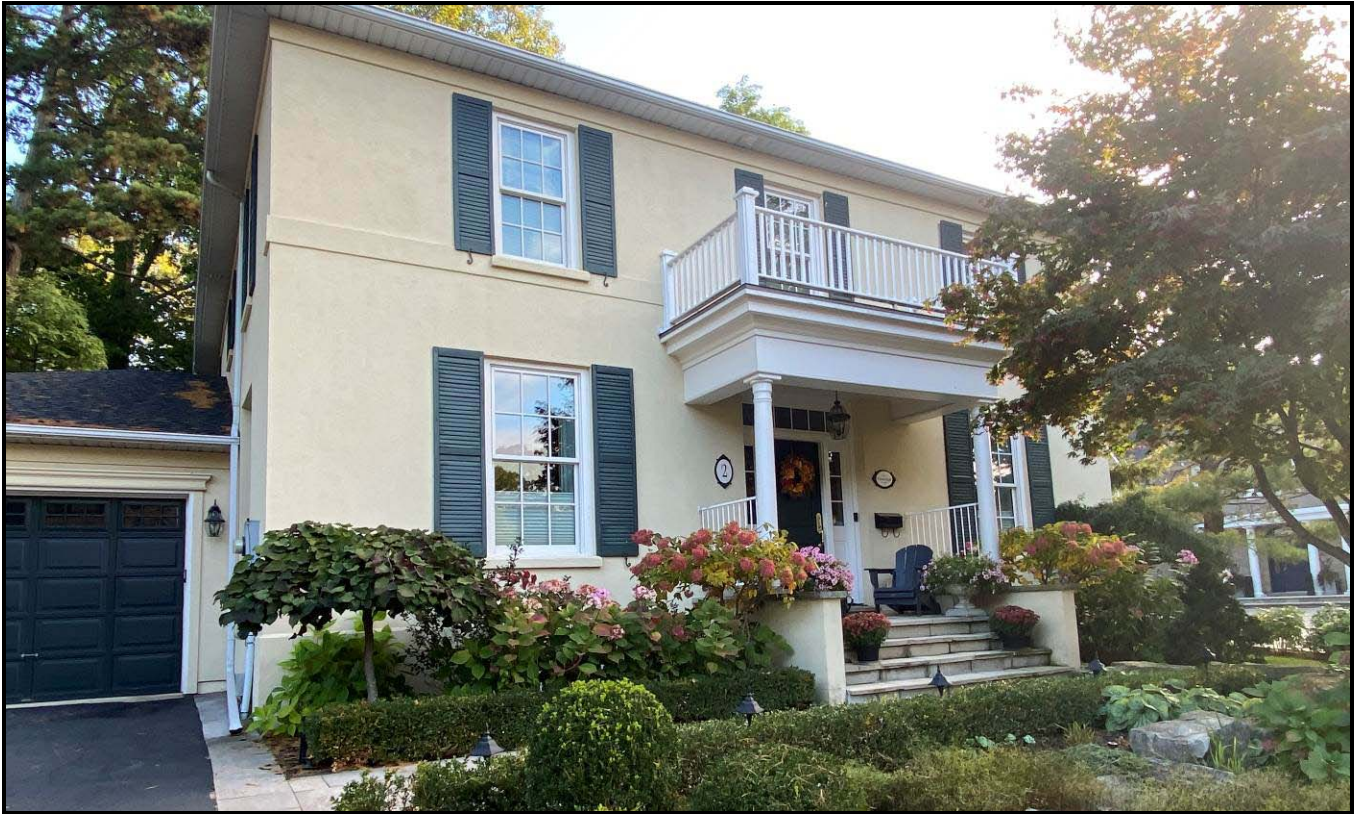
Front elevation of the subject house, 2023. The portico was rebuilt after the house was moved, and the brick was plastered over. The original house massing, fenestration, and elevation symmetry are still present. Source: Town of Oakville Planning Services staff
