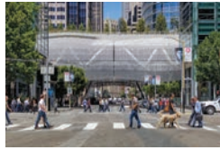
Salesforce Transit Centre and Park, San Francisco. Source: Salesforce Transit Centre
