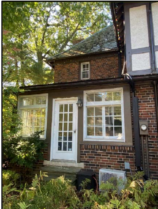
The east elevation sunporch. October 2023.
