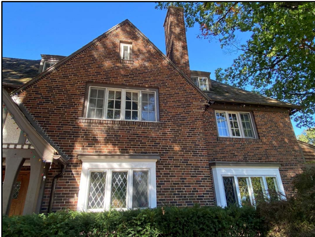
The house includes a variety of window styles and shapes. October 2023. Source: Town of Oakville, Heritage Planning staff photo
