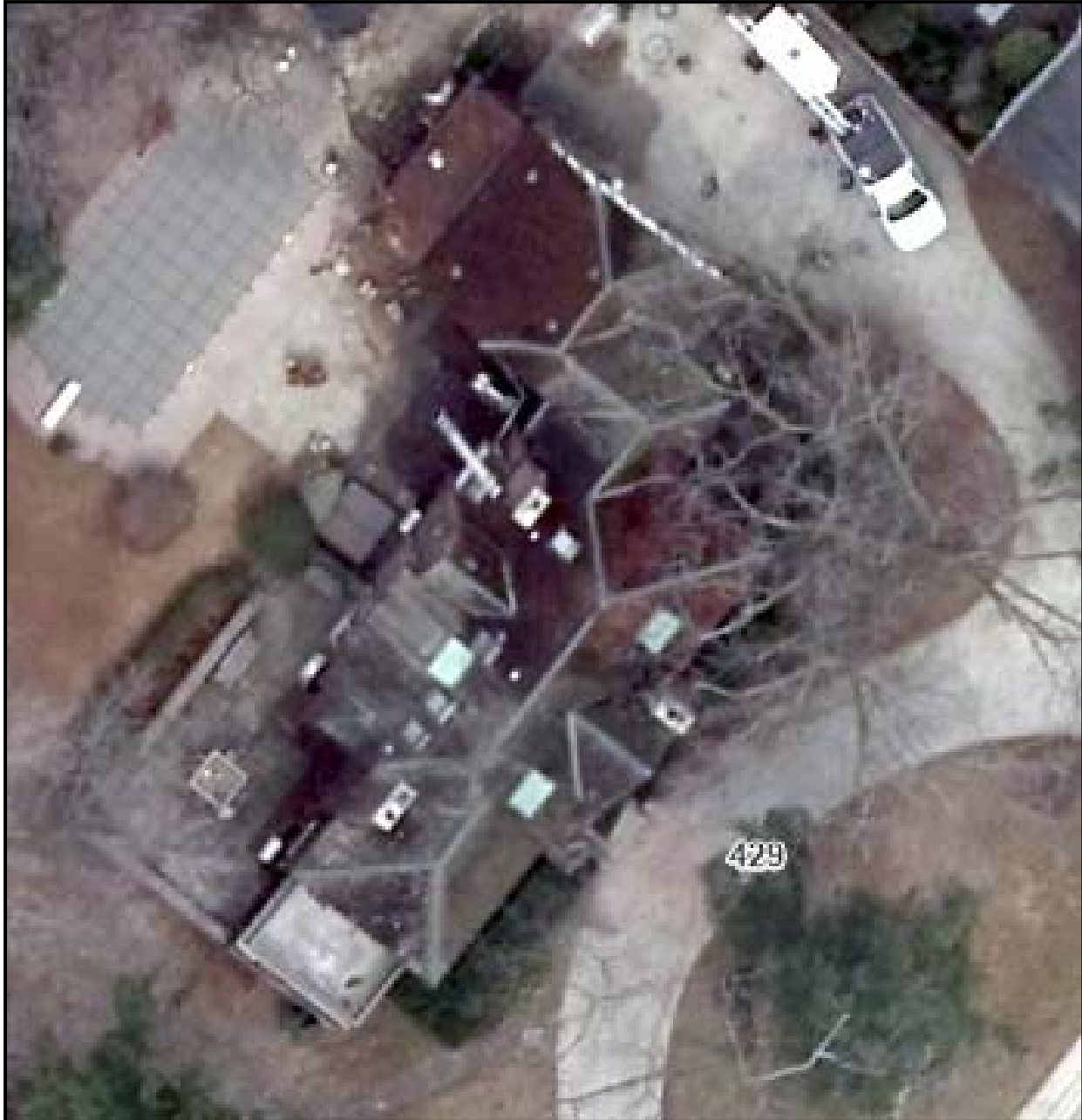
Aerial view of 429 Macdonald Road, showing its many sections. 2021
