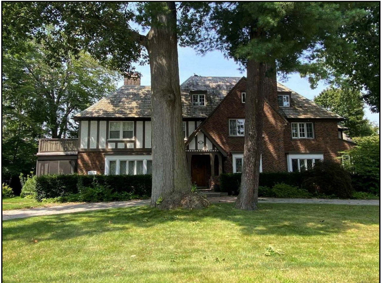
Front elevation of the subject house, August 2023
