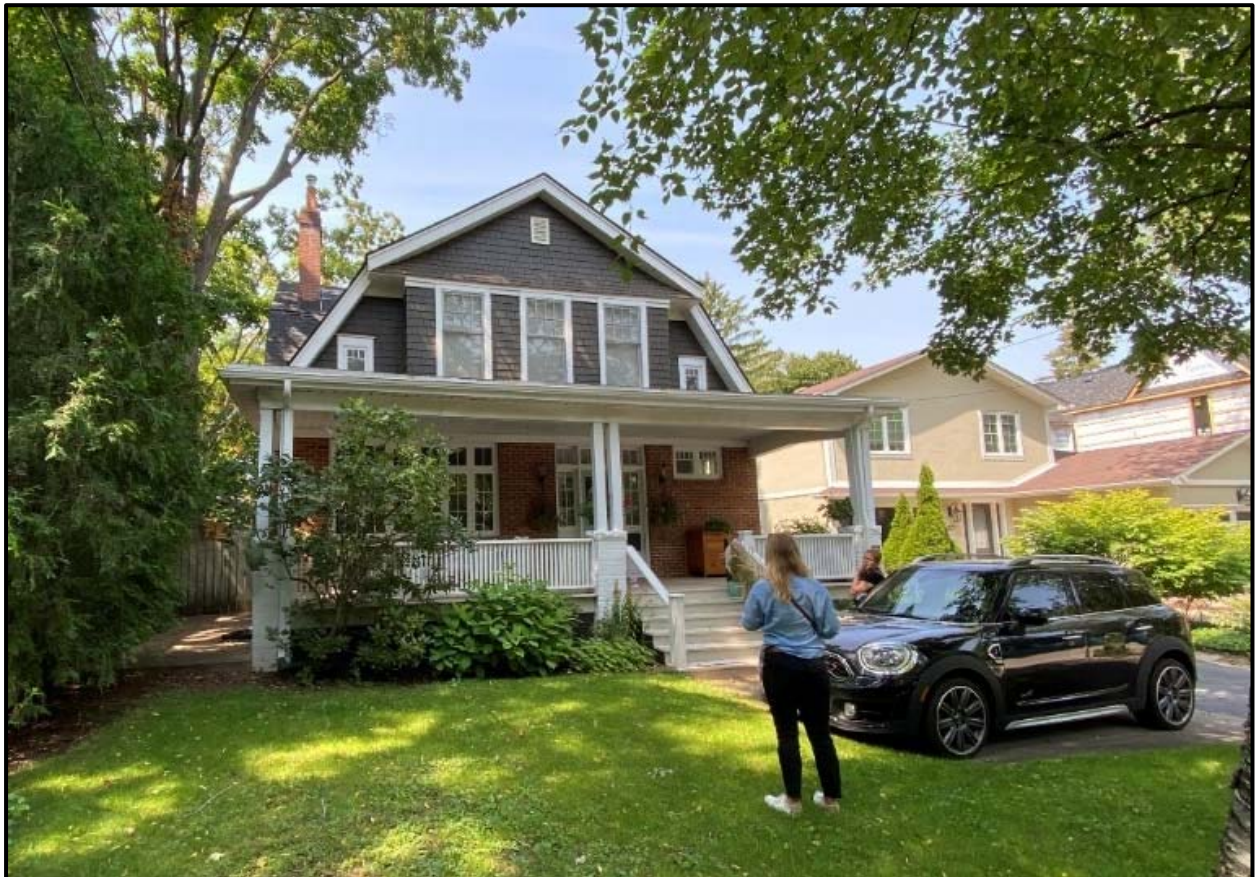
View of the southwest corner and front façade of the Cuthbertson House, August 2023
