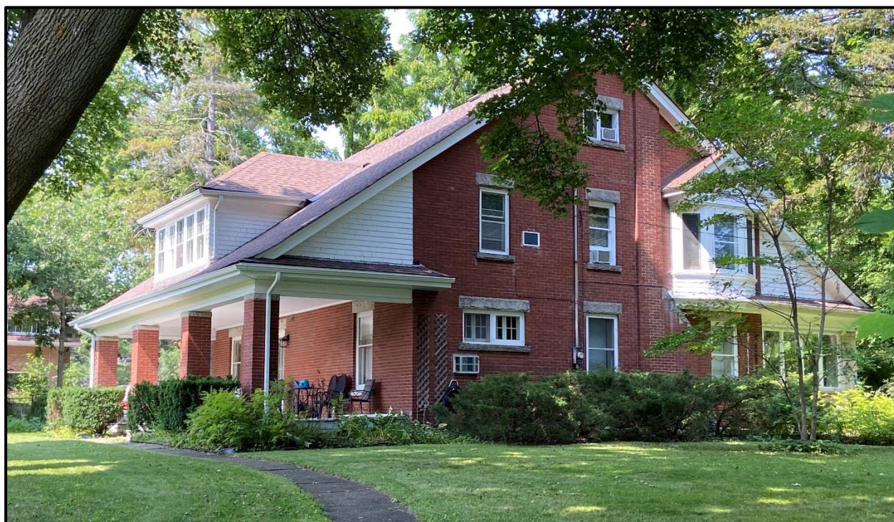
The original front façade of the Snyder House faces west toward Reynolds Street. Source: Town of Oakville, Heritage Planning staff photo
