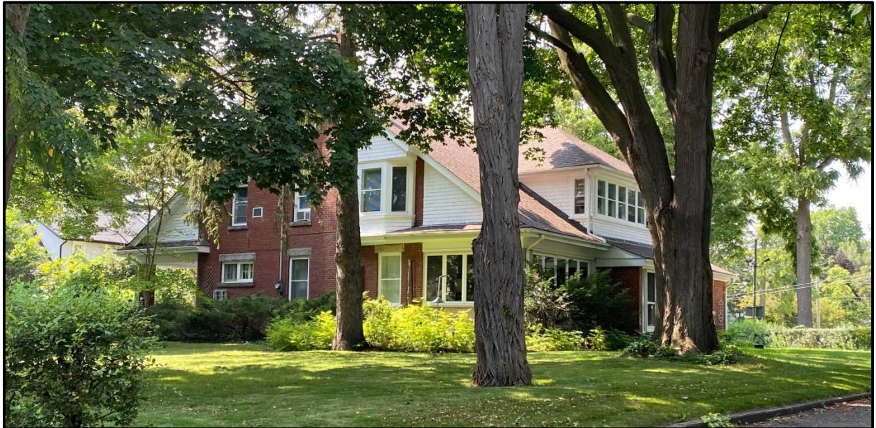
North-east corner of the Snyder House, August 2023
