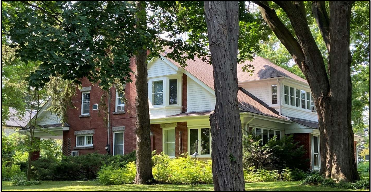
East elevation, showing some of the variety of windows used on the Snyder House. Source: Town of Oakville, Heritage Planning staff photo
