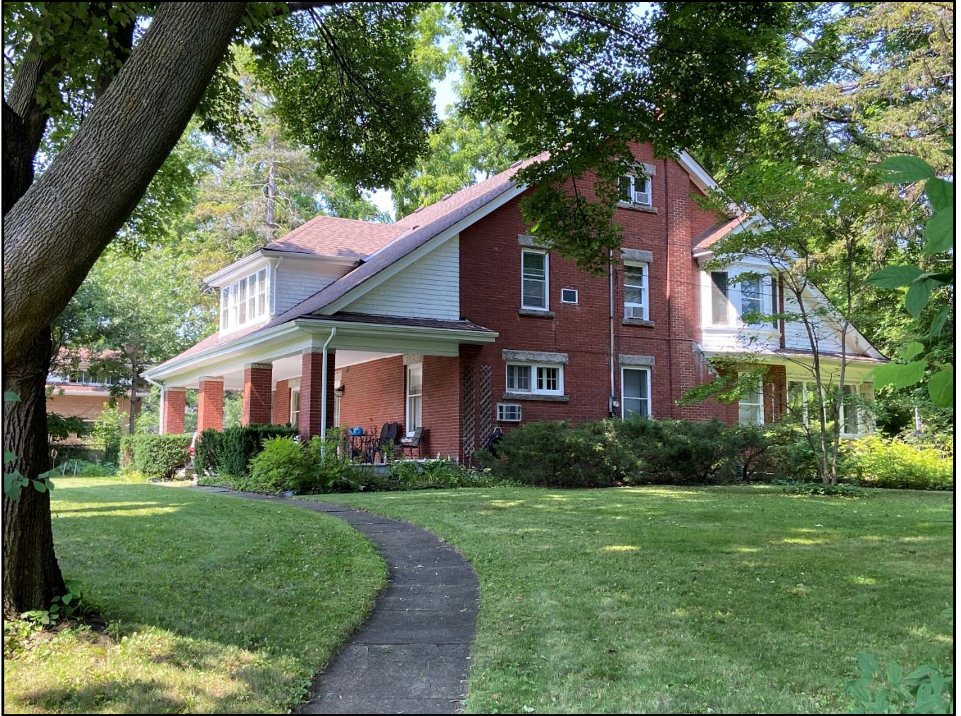
The Snyder House, August 2023. Source Town of Oakville Planning Services Staff
