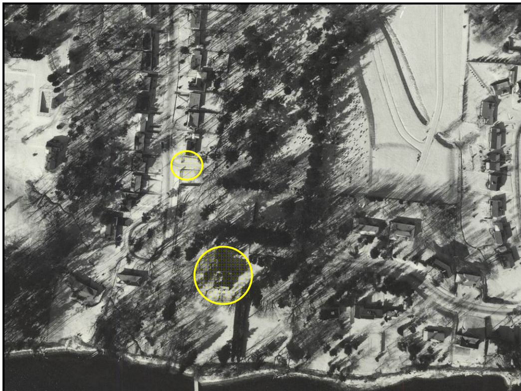
1962 aerial photo of historical Lot 17. The earlier subdivided western portion is now built on, as well as the small square section to the east, which was subdivided in the 1950s. The historic house is the large yellow circle, and the pillars and their second location are in the smaller circle. 45 Source: McMaster University Library, Queen Elizabeth Way and Highway 2 Corridor
