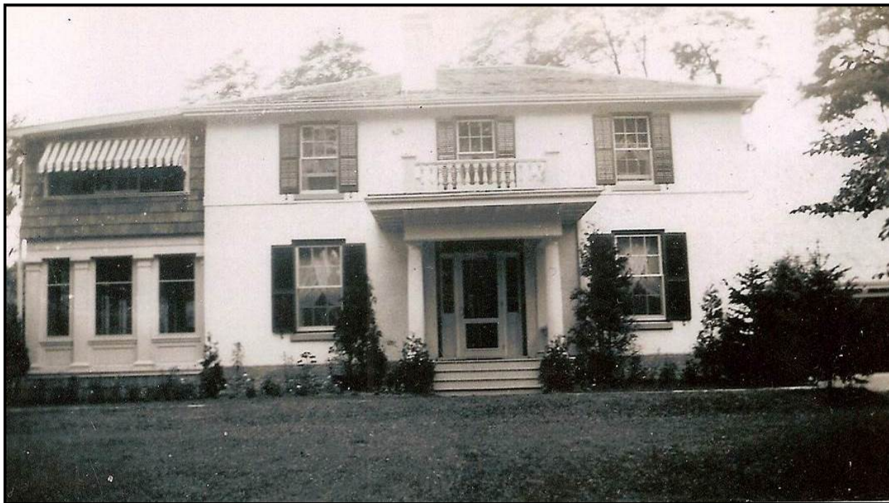
The front of the house during the Lefebvre ownership. The house had been painted, and the south porch built by the Stuarts was enclosed, with the upper floor extension covered in cedar shingles. Source: Trafalgar Township Historical Society, TTHS003235536f
