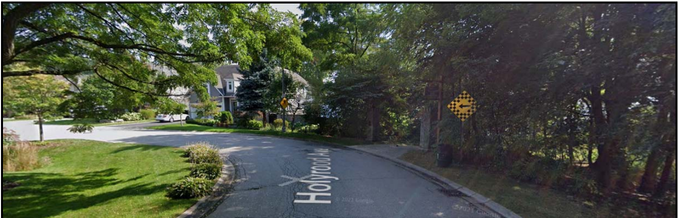
View of the pillars looking south on Holyrood Avenue, to the right. Source: Google Street View
