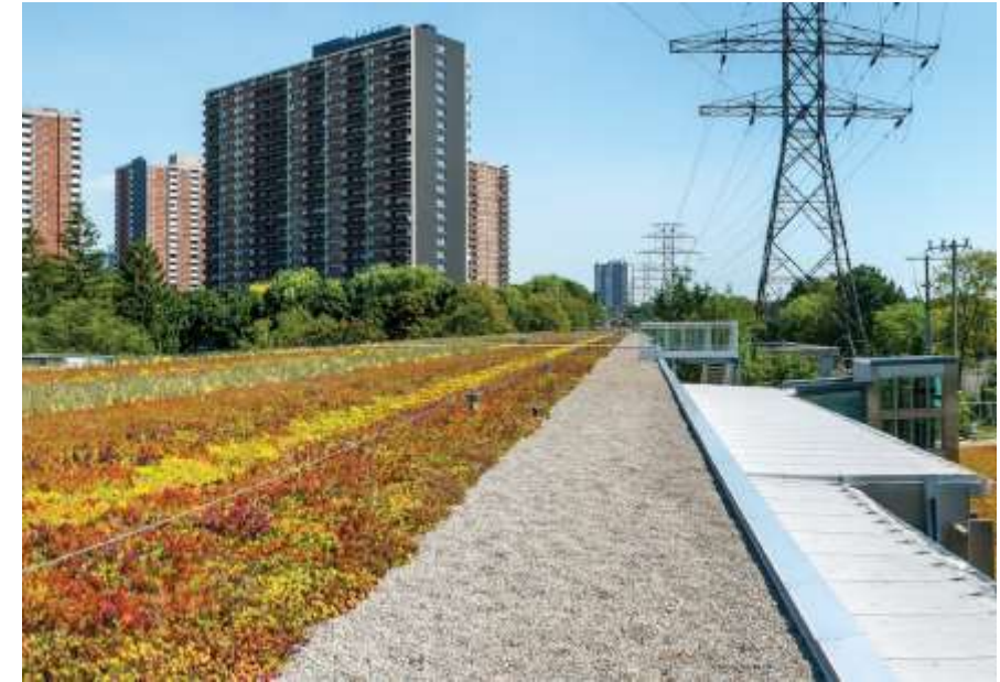
Green roof atop ESRI Canada, photo by Scott Source: Torrance Landscape Architect Ltd.
