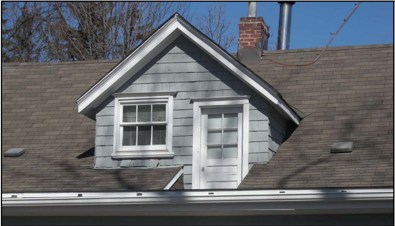
Close up of the door and window in the west dormer, 2010. The window is 3/3. Source: Source: Town of Oakville Planning Services Staff
