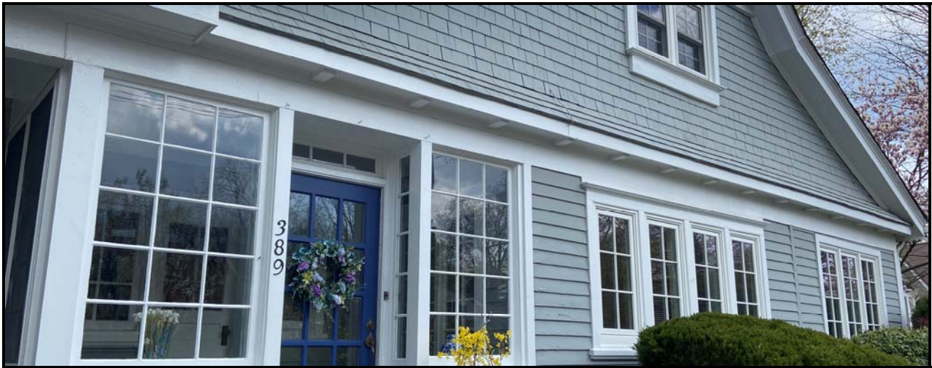
Bell-cast overhang and exposed eaves on the south elevation of the house. Source: Town of Oakville Planning Services Staff
