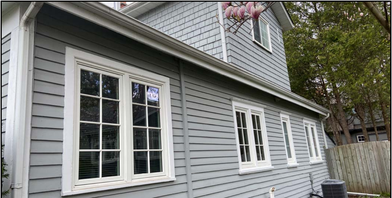
West elevation of the home showing casement windows on the first floor and the updated dormer. Source: Town of Oakville Planning Services Staff
