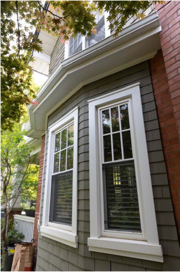
View of the north elevation showing the first storey bay window. Source: Town of Oakville Planning Services Staff
