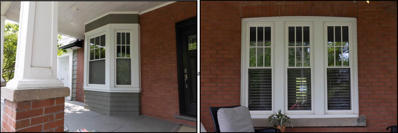
Close up of the window styles on the front porch; bay window on the south side and three row 6/1 on the north. A row of three windows on the front porch is often seen in Craftsman houses. Source: Town of Oakville Planning Services Staff
