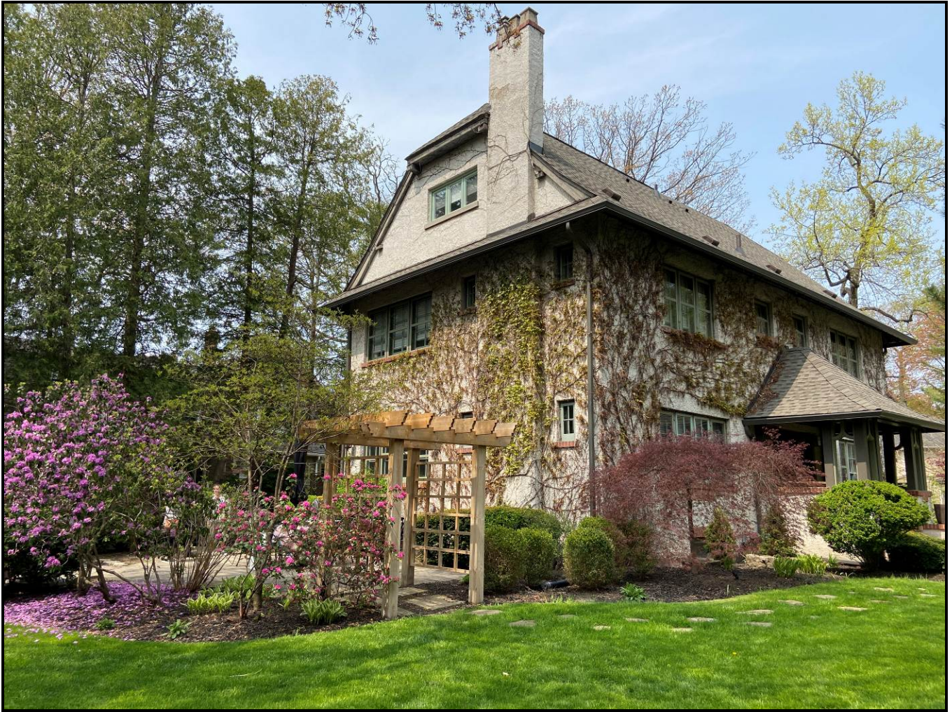
West elevation, facing the backyard, with some of the south elevation. Source: Town of Oakville Planning Services Staff
