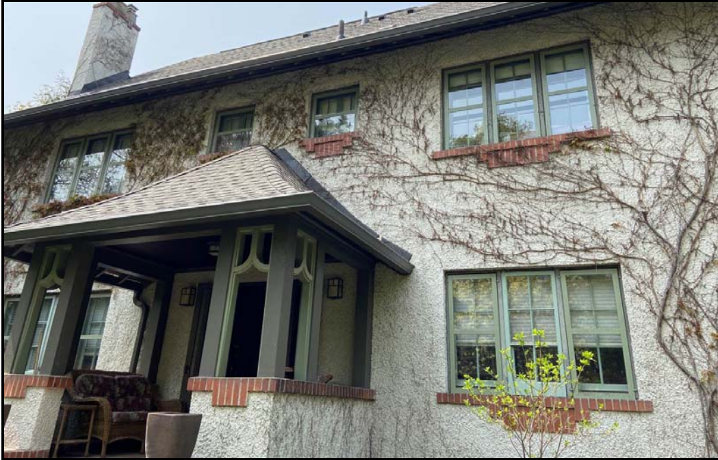
South elevation, east side, showing six pane windows and four panes above the porch. Source: Town of Oakville Planning Services Staff
