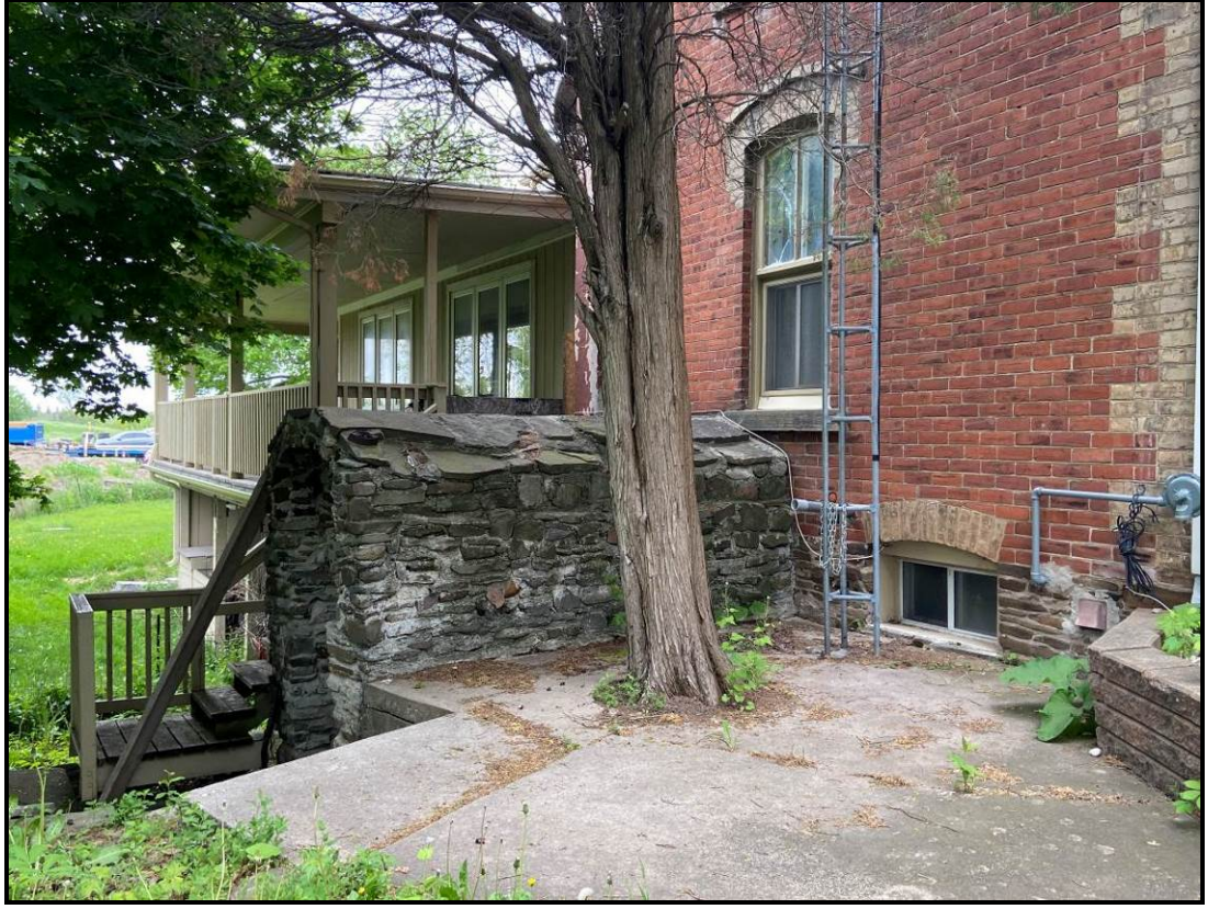
South façade detail:
