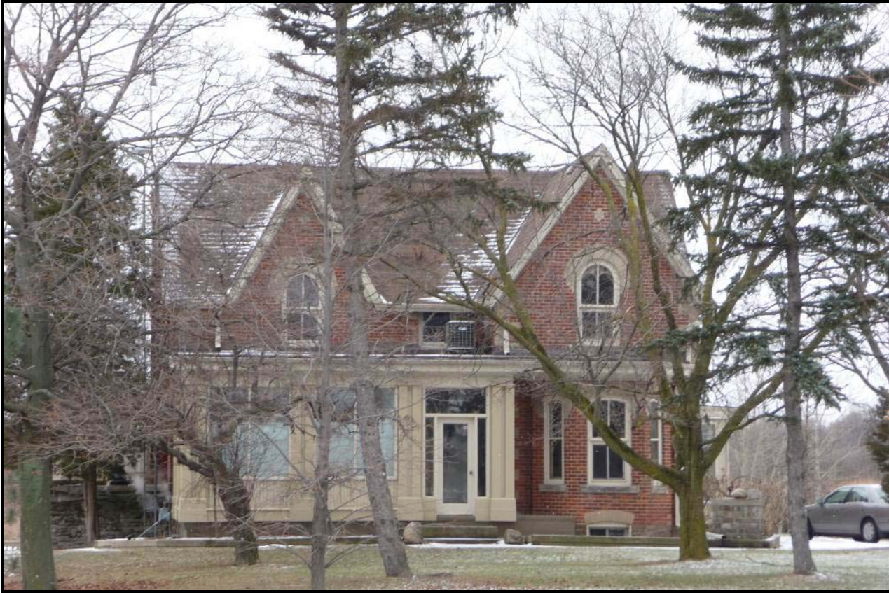
3480 Ninth Line, December 2008 Source: Planning Services photo
