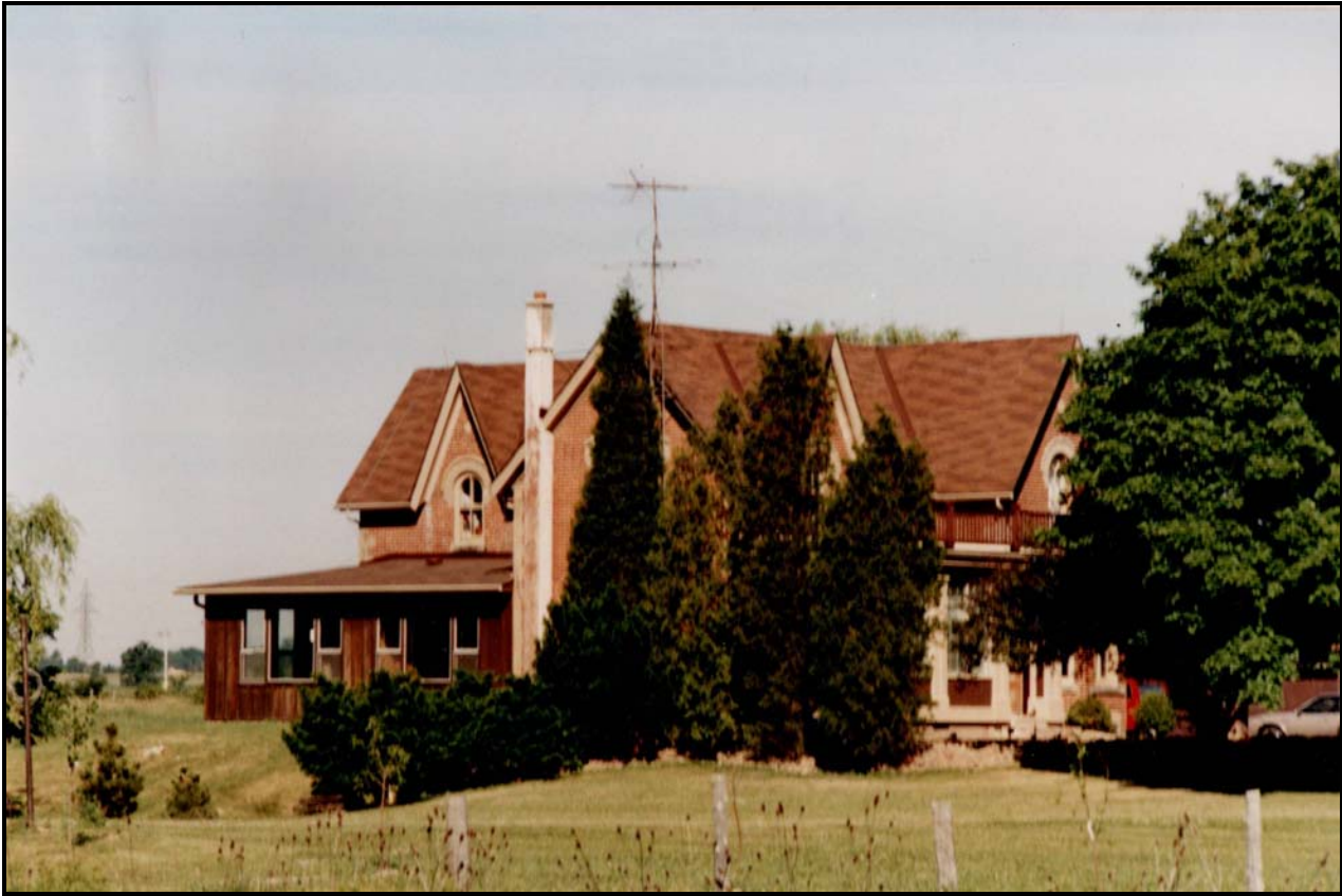
c.1991 photo of the south and east elevations. Note the enclosed front porch. Source: Town of Oakville Planning Services staff photos
