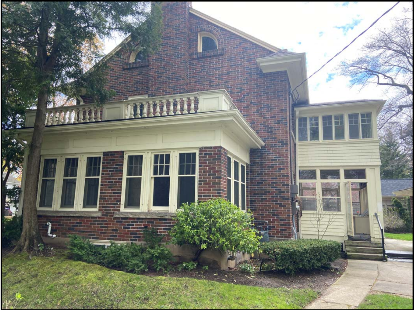
East elevation of the home at 405 Galt depicting several heritage elements, such as the second storey porch balustrades and quarter lunette windows. Source: Town of Oakville Planning Services Staff
