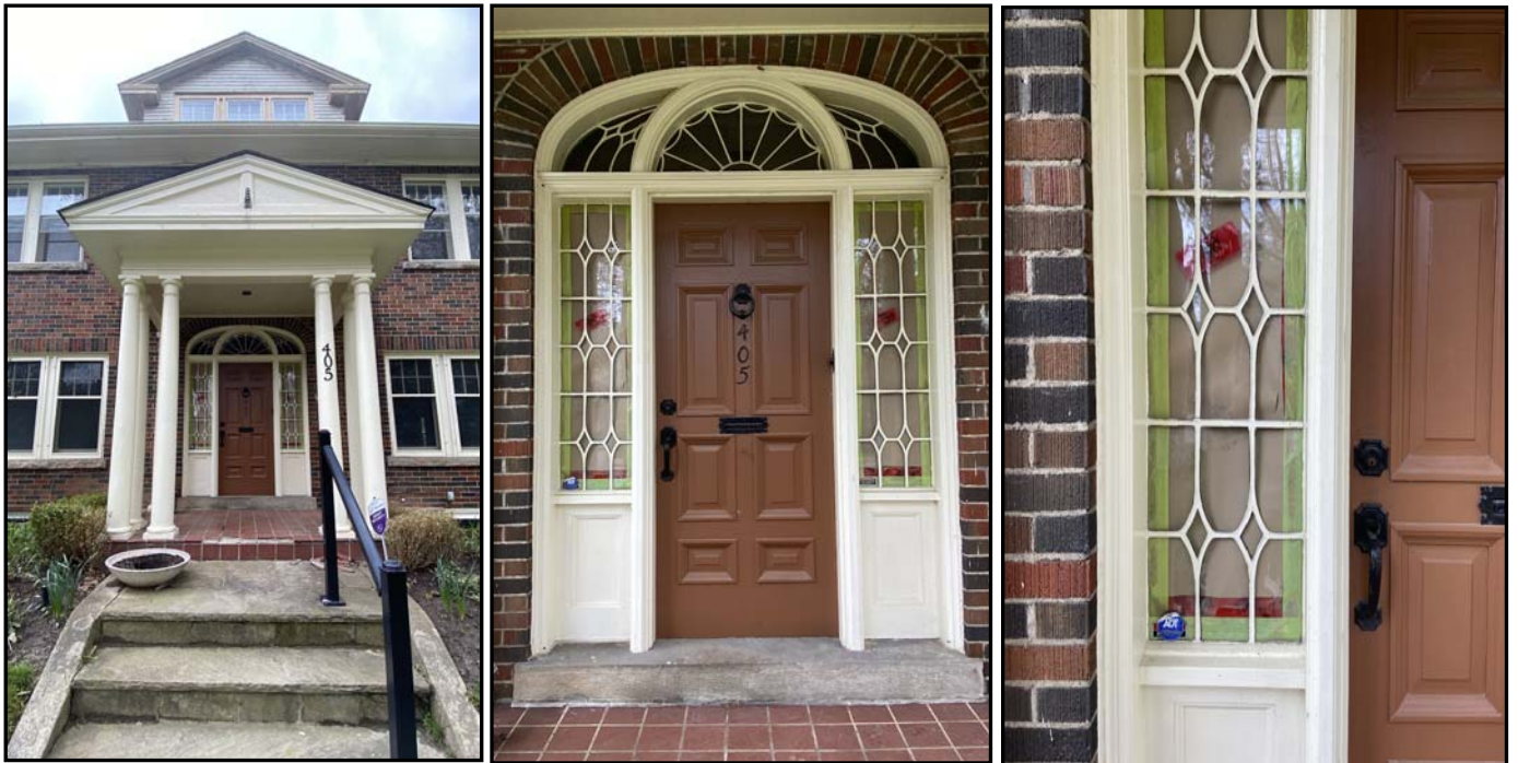
Front of the home showing symmetrical façade and the porch columns, pilasters, and the window design around the front door. Source: Town of Oakville Planning Services Staff
