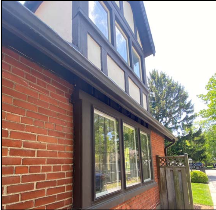
One example on the house where two sets of three-row windows can be seen, north elevation, 2023. Source: Town of Oakville Planning Services Staff
