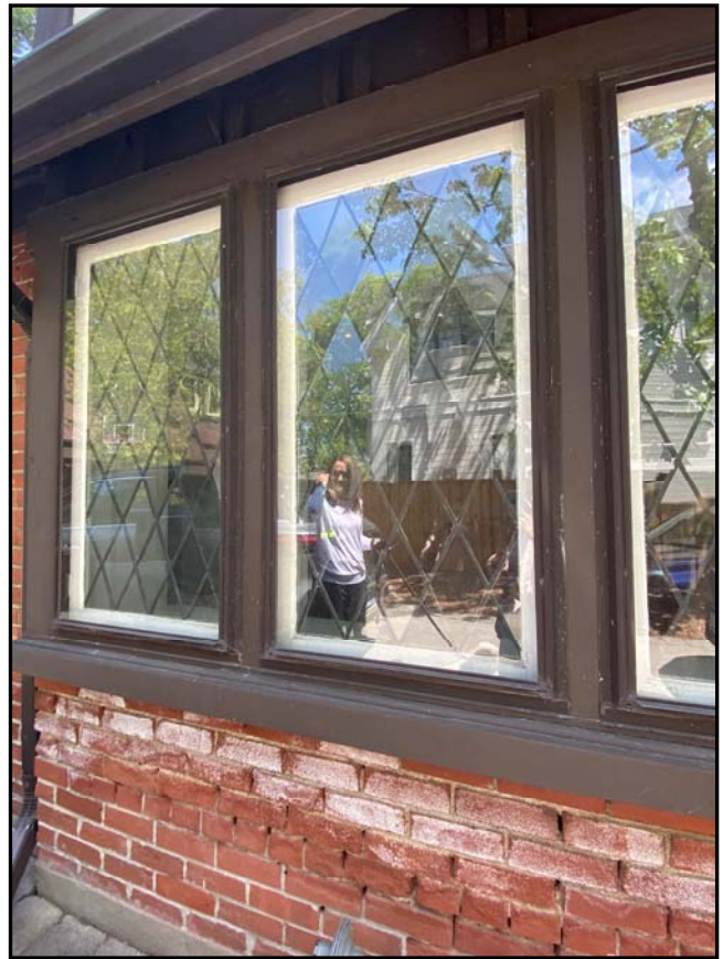
Close ups of some of the windows showing the diamond pattern and wooden casements and sills under the newer storm windows, 2023. Source: Town of Oakville Planning Services Staff
