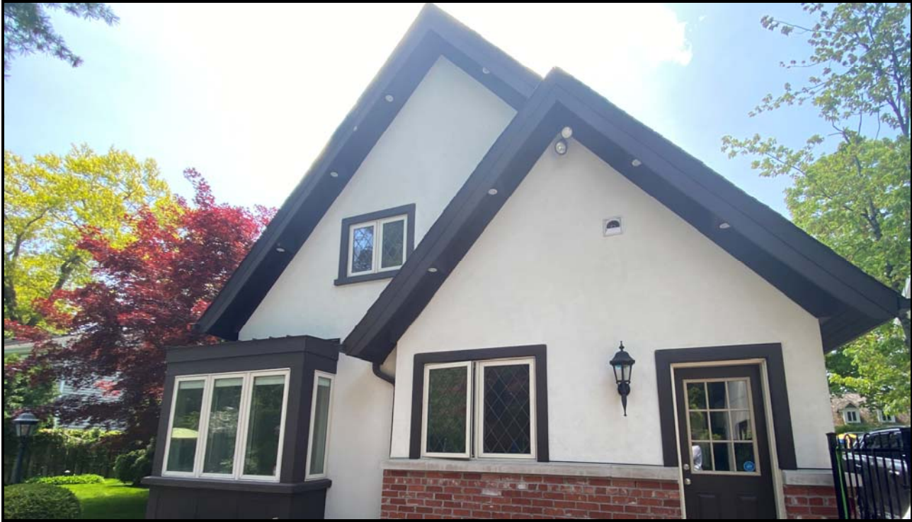
Rear addition, 2023. Source: Town of Oakville Planning Services Staff
