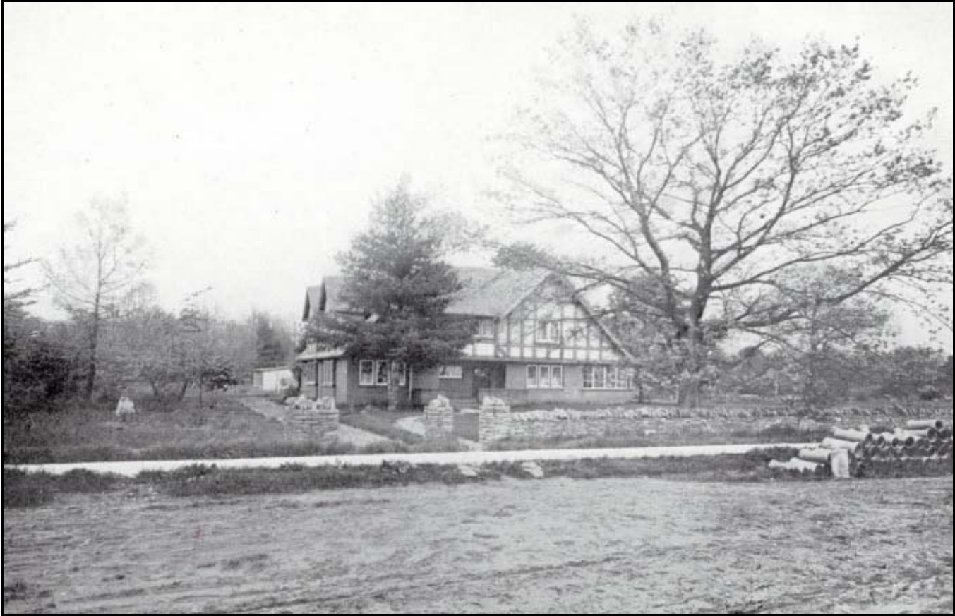
1913 image of the house, showing original elements that still stand such as the lakestone wall and columns, the cladding of the house, and its fenestration. Source: 1913 Brantwood promotional booklet, Cumberland Land Company Ltd. and W.S. Davis
