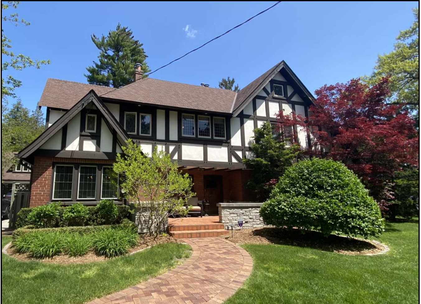
West elevation (front) of the house, 2023. Source: Town of Oakville Planning Services Staff
