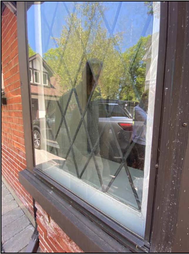
Close ups of some of the windows showing the diamond pattern and wooden casements and sills under the newer storm windows, 2023. Source: Town of Oakville Planning Services Staff
