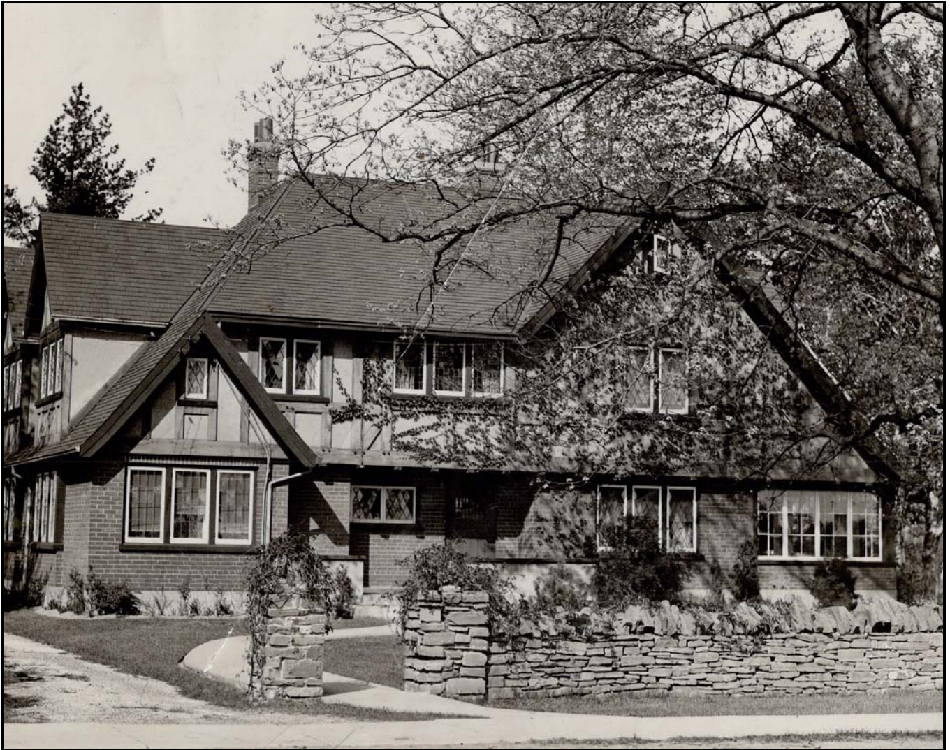
Photo of the house in 1929, published in the Toronto Star. One can see that several original elements are still intact, such as the half-timbering and the low lake stone knee wall. Source: Toronto Public Library – Toronto Star Photograph Archive
