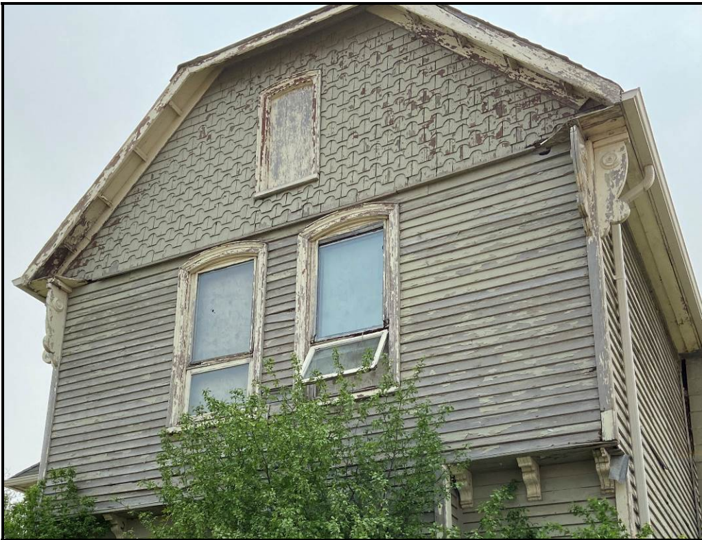
Close-up of the jerkinhead gable with decorative cedar shingles, exposed eaves, wood corbels, segmentally arched windows and bracketed frieze below second storey. May 2023. Source: Town of Oakville, Heritage Planning staff photo
