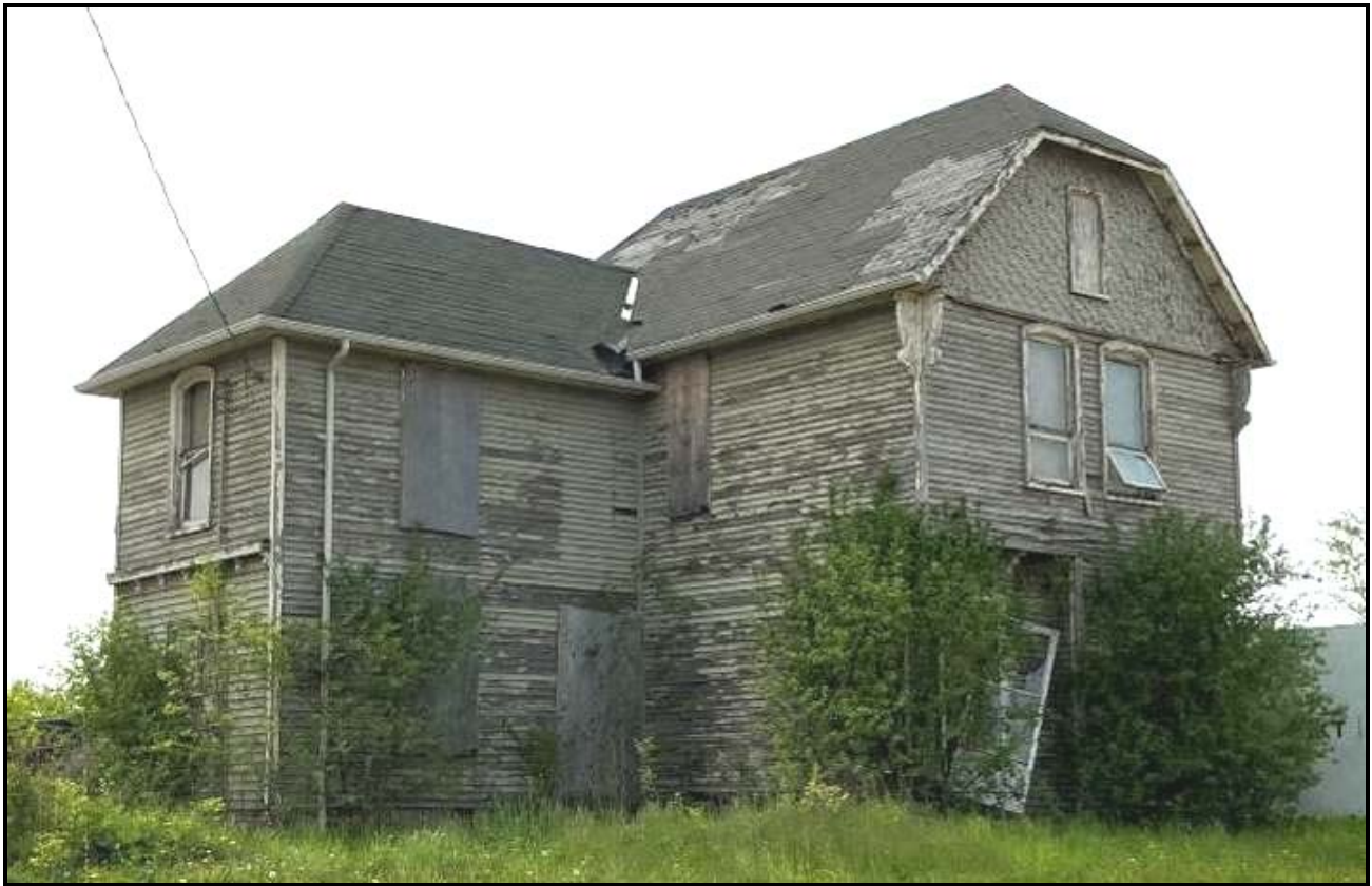
South (side) and east (front) elevations of the house. Decorative wood friezes with brackets remain intact on both elevations. May 2023. Source: Town of Oakville, Heritage Planning staff photo
