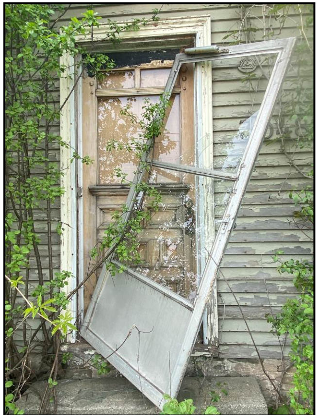
Close-up view horizontal wood siding and wood corner board trim; close-up of the original front door behind a contemporary metal screen door. May 2023. Source: Town of Oakville, Heritage Planning staff photo
