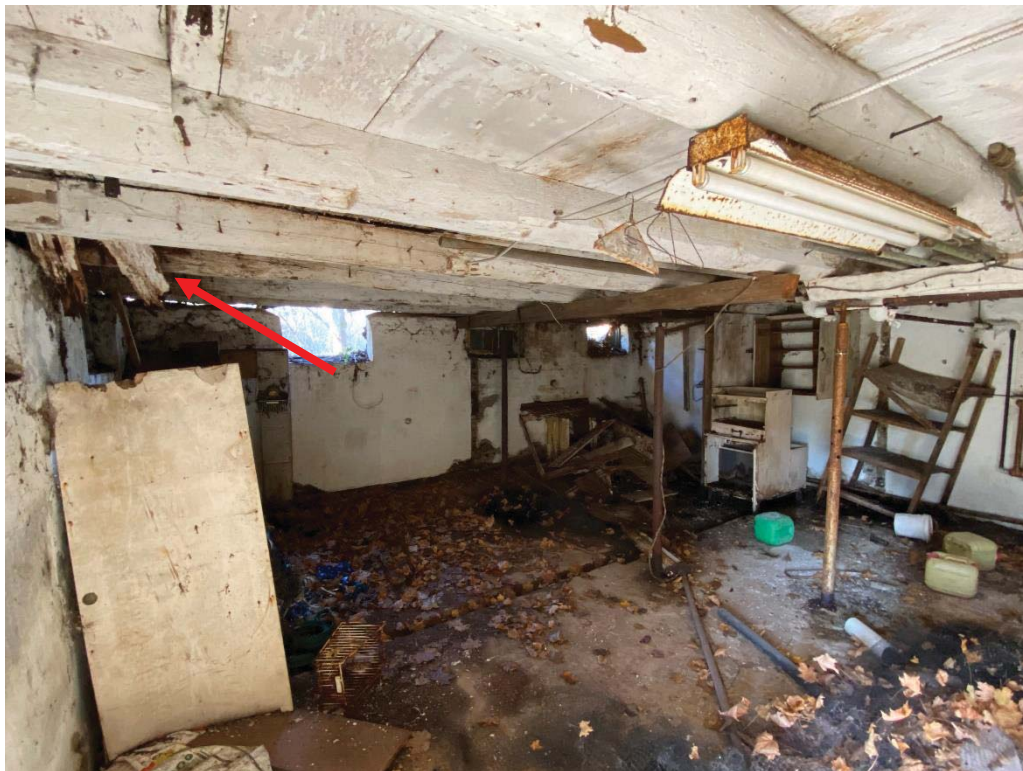
Photograph No. 15 – Stained and Rot Basement Roof Wood Beams
