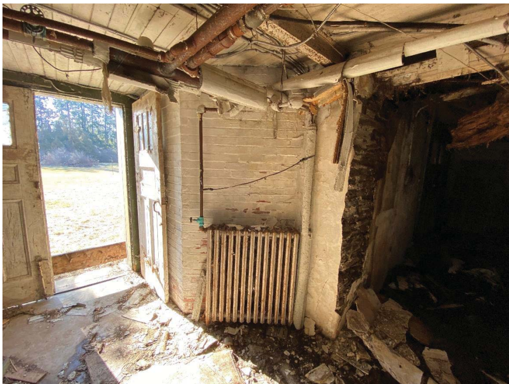
Photograph No. 10 – Basement Stone and Brick Foundation Walls
