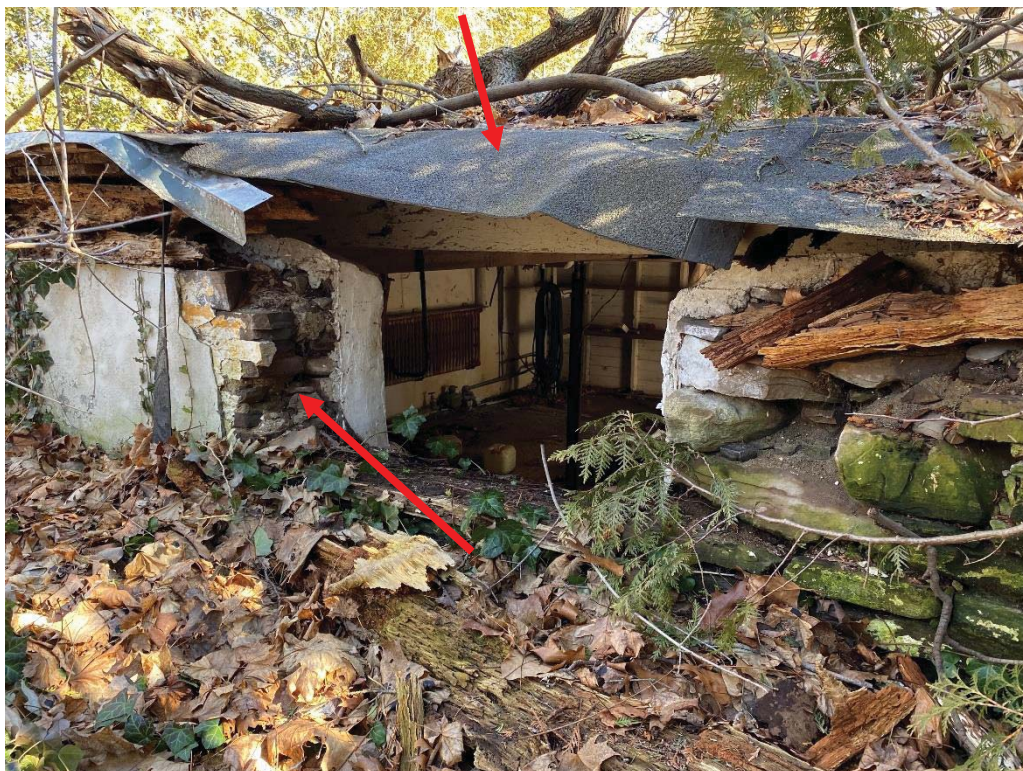
Photograph No. 6 – Deteriorated Basement Roof and Stone Foundation Walls
