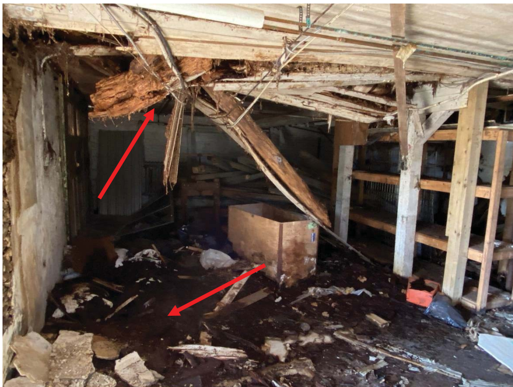
Photograph No. 13 – Evidence of Water in Basement; Collapsed Basement Roof
