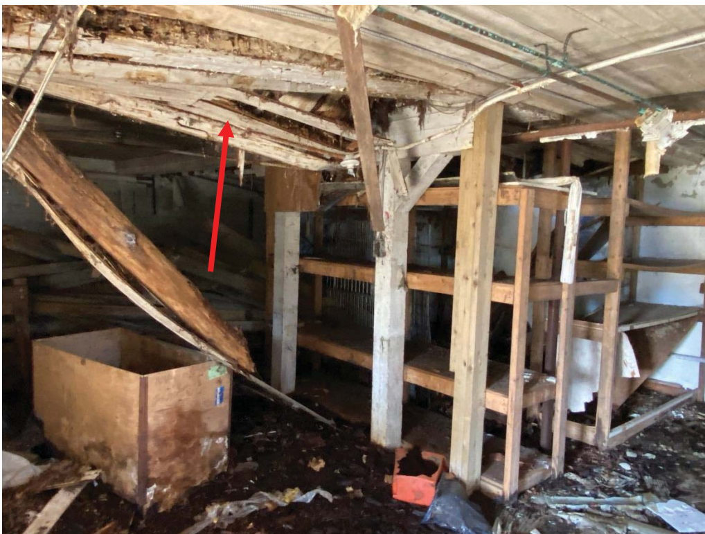
Photograph No. 12 – Collapsed Basement Roof Structure
