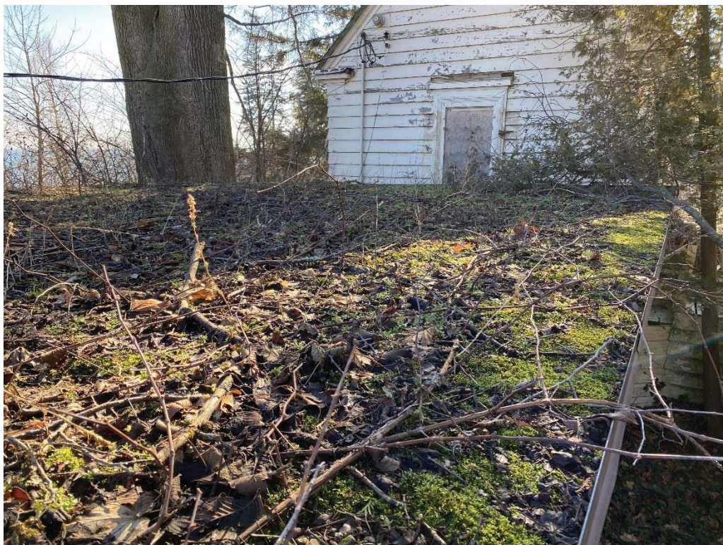
Photograph No. 20 – Garage Roof; Vegetation Growth
