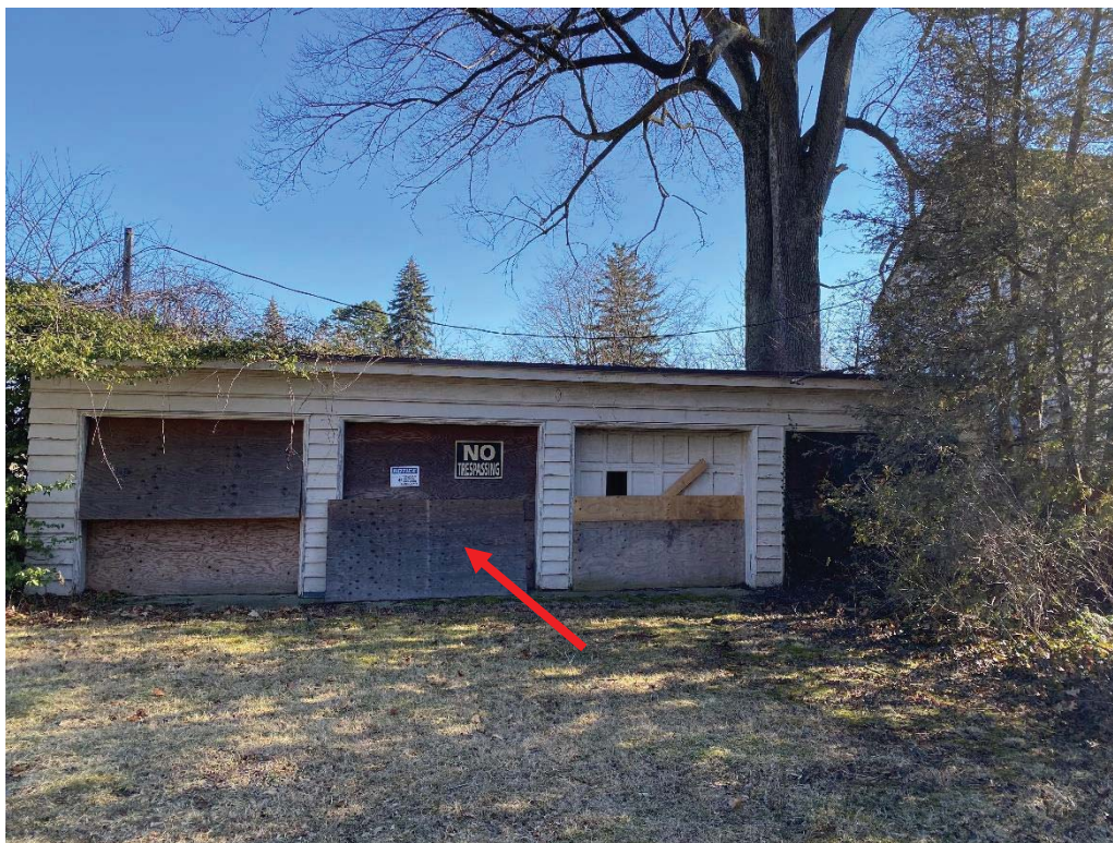
Photograph No. 3 – Garage Front Elevation – Deteriorated Building Envelope and Boarded Up Doors
