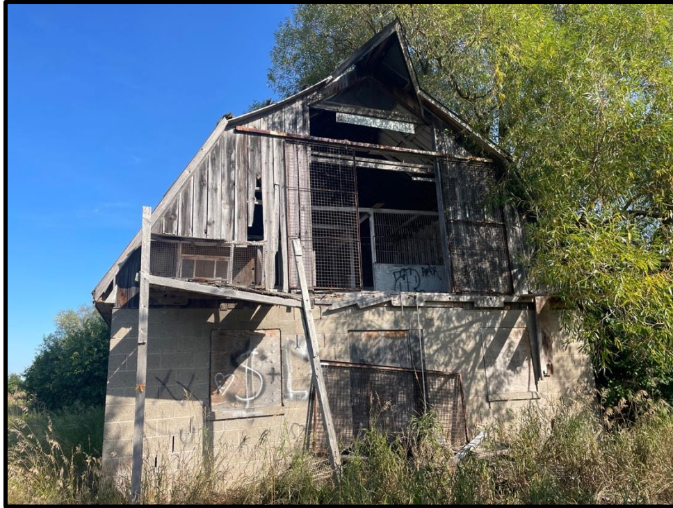
Image 5: 2165 Dundas Street West – East Elevation (Photo taken August 18, 2022; Facing Northwest)
