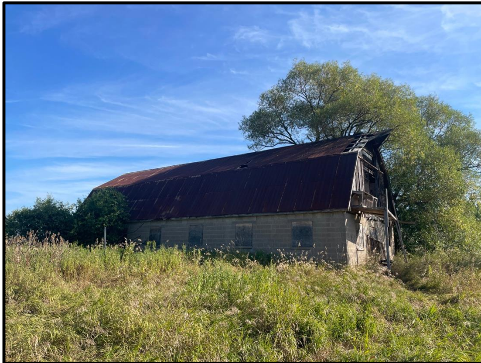
Image 6: 2165 Dundas Street West – South Elevation (Photo taken August 18, 2022; Facing North)
