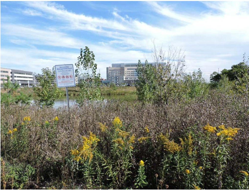
Figure 12: View of new Oakville Hospital and research buildings to the east, with storm water pond in foreground. (AB, 2015)
