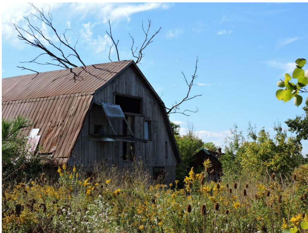
Figure 10: Rear (north elevation) of barn with shed in background. (AB, 2015)
