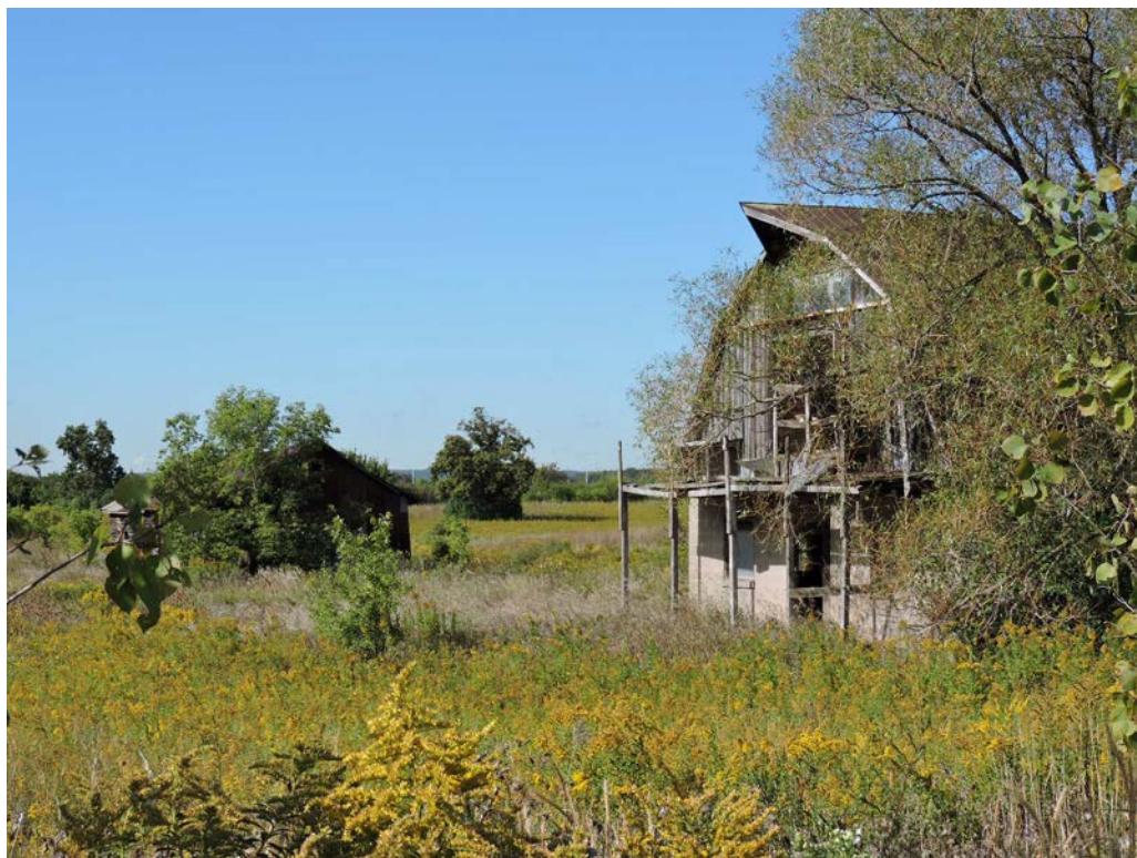
Figure 9: View of barn with shed in background. (AB, 2015)
