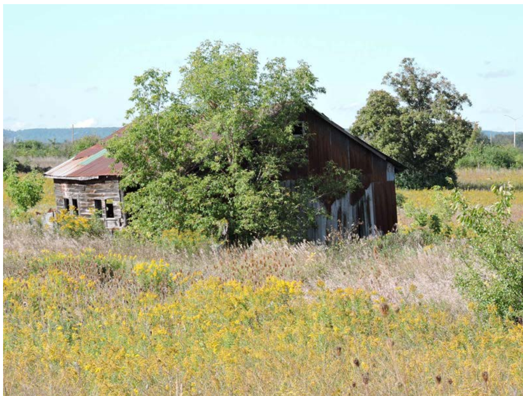
Figure 7: Detailed view of shed. (AB, 2015)
