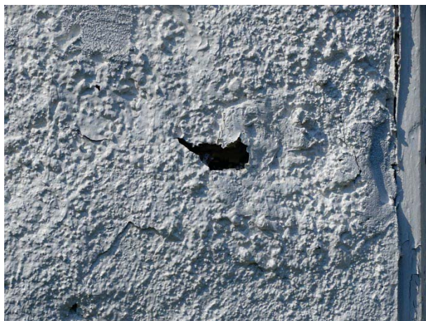
Figure 63: Exterior stucco detail showing small hole
