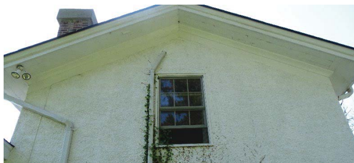
Figure 65: Fascia Detail with aluminum downspout
