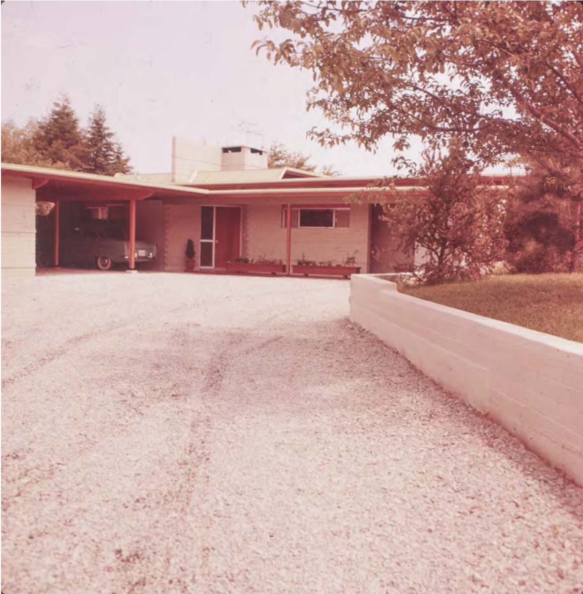
FRONT ENTRANCE – the window on the main elevation has been enlarged and the car port has been enclosed
