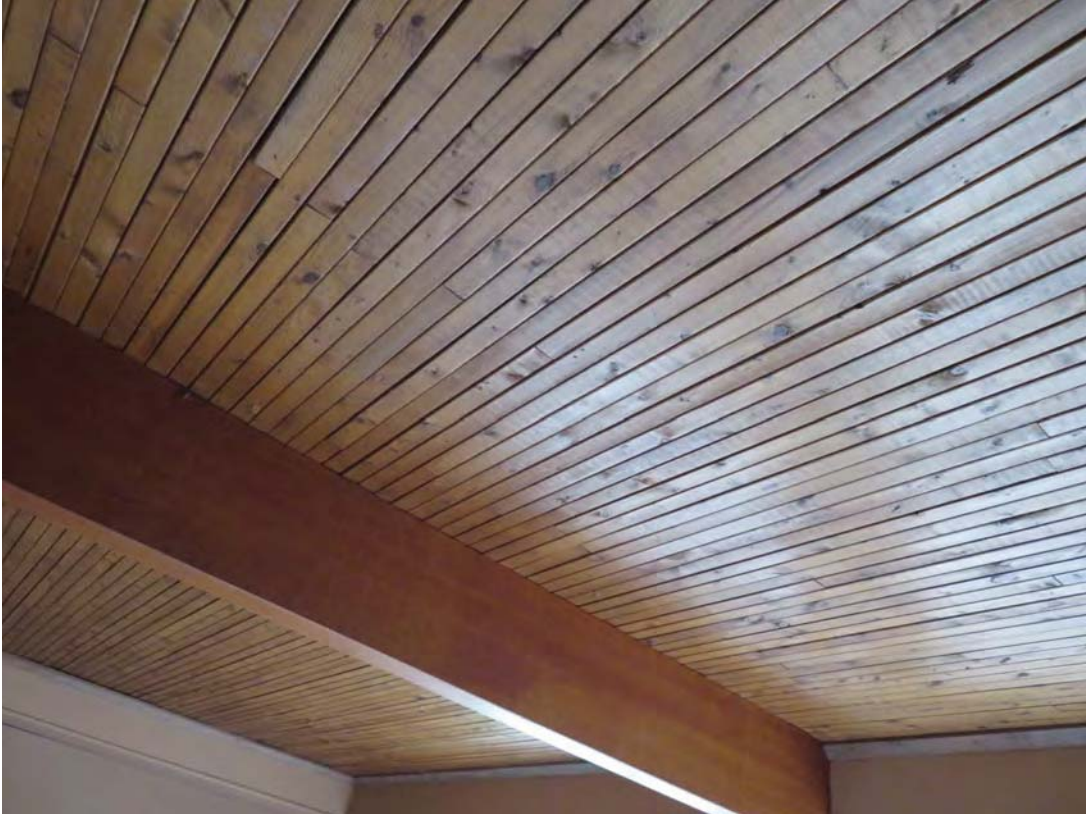
STRUCTURAL WOOD BEAM AND WOOD CEILING
