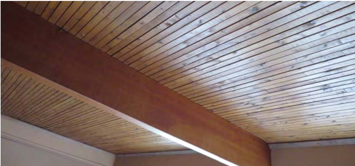
POTENTIAL SALVAGE ITEM: wood ceiling beams
