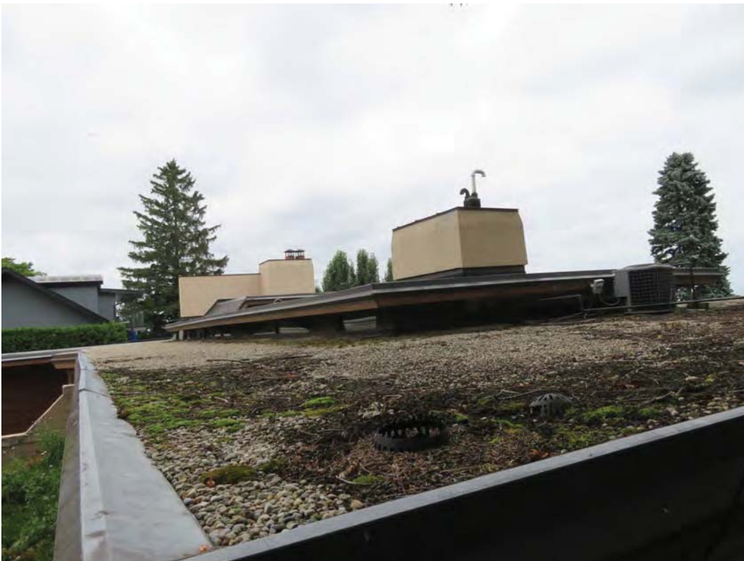
ROOF – gravel roof with organic debris and biological growth
