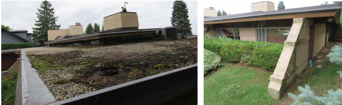
CONDITION ISSUES: organic growth on the roof and masonry indicating persistently wet conditions
