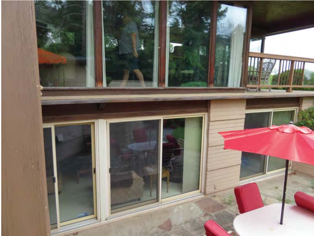
SIDE ELEVATION – original glazing has been replaced on the lower level
