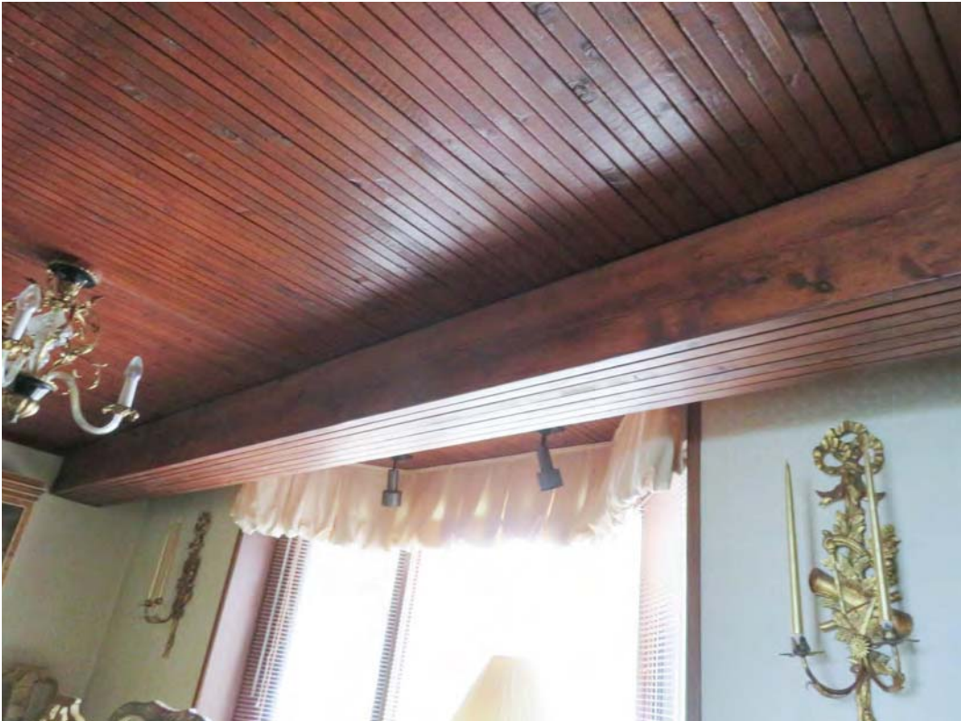
LAMINATED WOOD BEAMS AND WOOD CEILING
