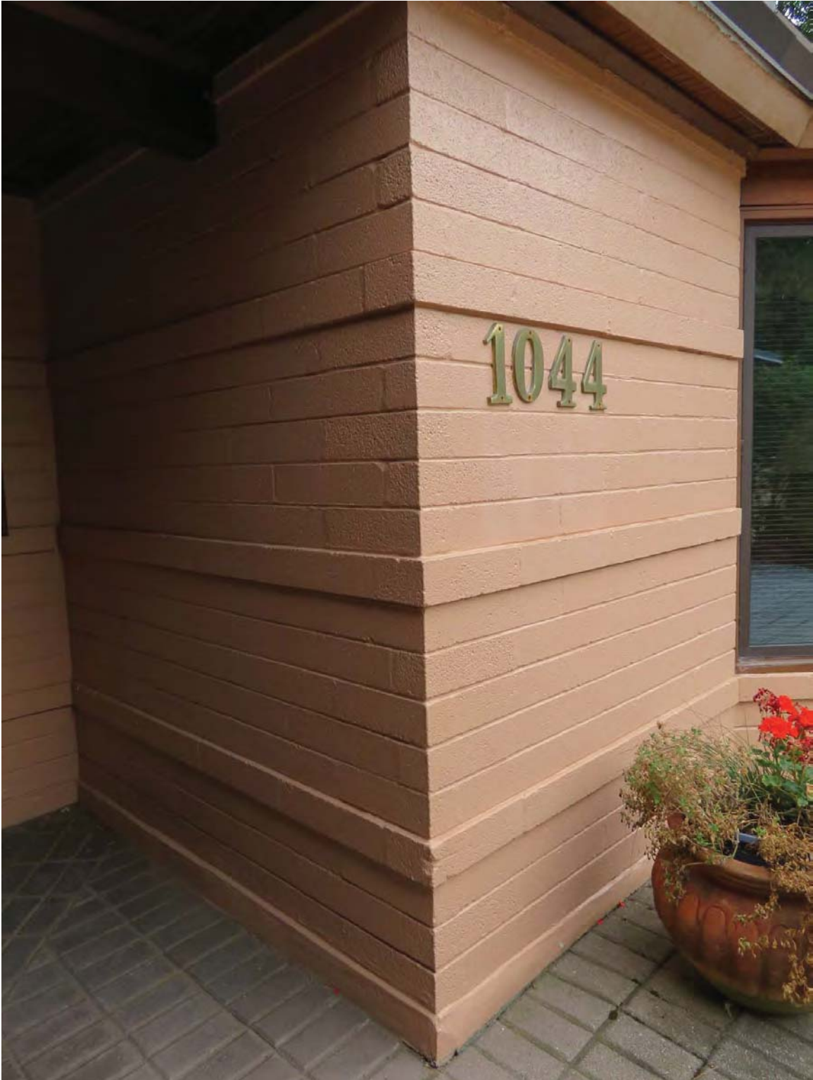
FRONT ELEVATION – masonry detail – horizontal banding
