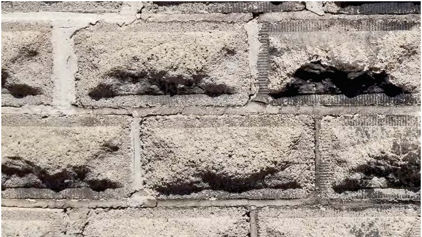
Figure 71 Rock-face CMUs with tooled edge
