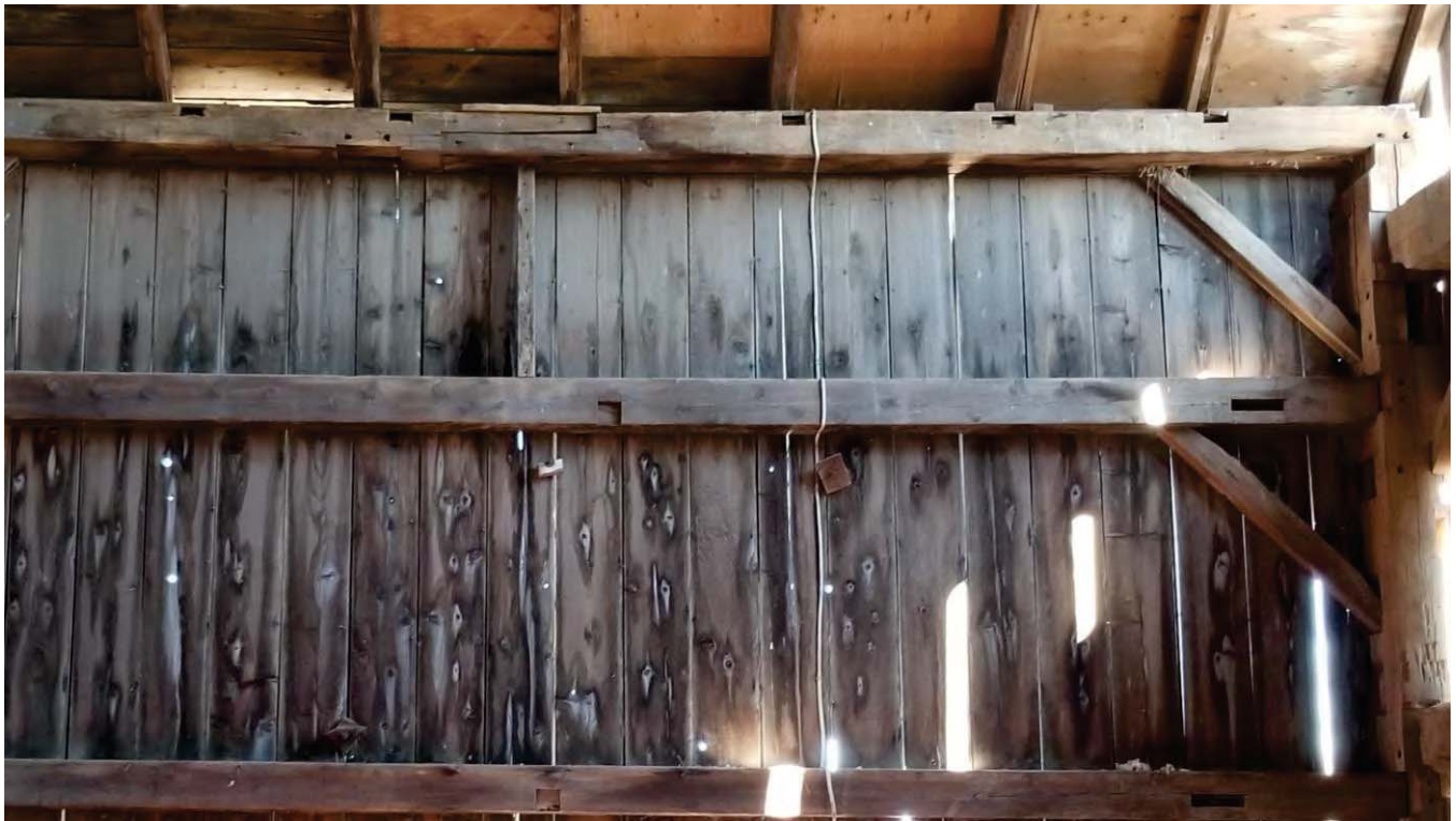
Figure 90 Posts, grits, and plate showing evidence of redundant mortices and treenail holes.
