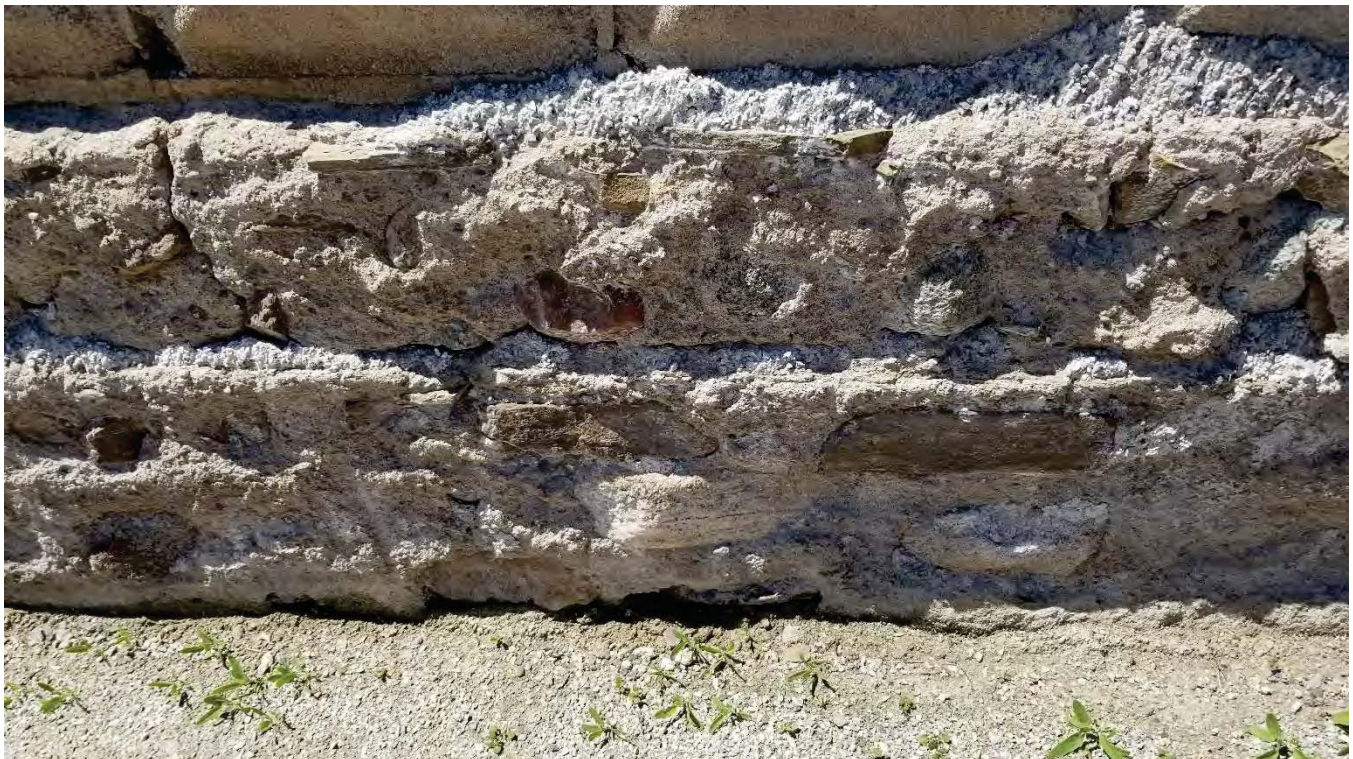
Figure 70 Coursed rubble stone foundation of the barn.
