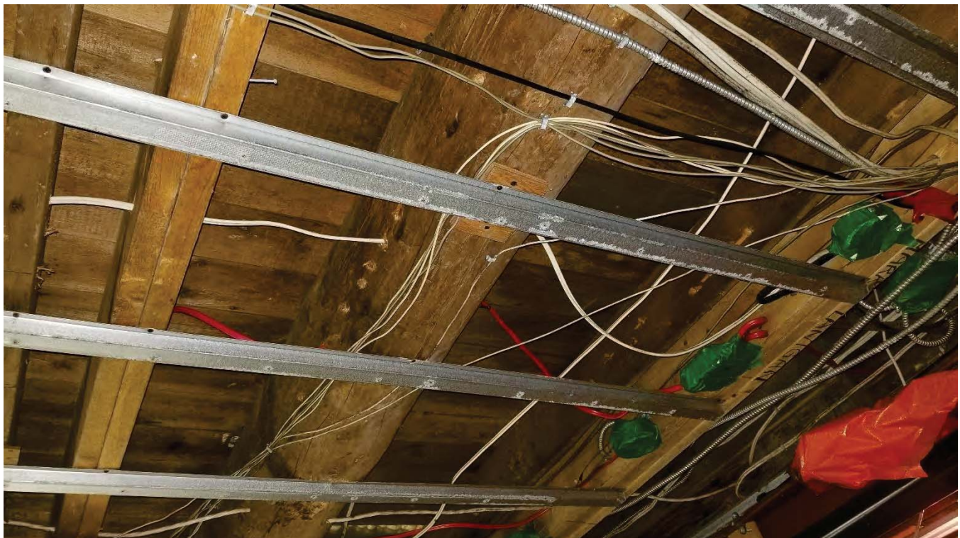
Figure 54 Basement, round timber and dimensional joists.
