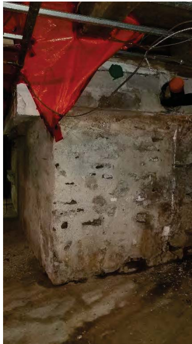
Figure 39 Basement looking north at raised foundation and opening to the left where the northwest foundation wall was cut and remove to join the basement of the rear extension.
