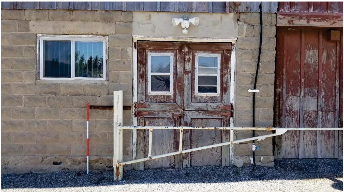
Figure 74 Double-leaf Dutch door in timber with one-over-one single hung windows and a concrete lintel on southeast elevation of the barn.
