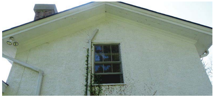
Figure 65: Fascia Detail with aluminum downspout
