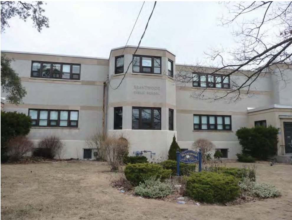
EXTERIOR – FRONT ELEVATION – STUCCO WITH HORIZONTAL STONE BANDING – PAINTED BRICK FOUNDATION
