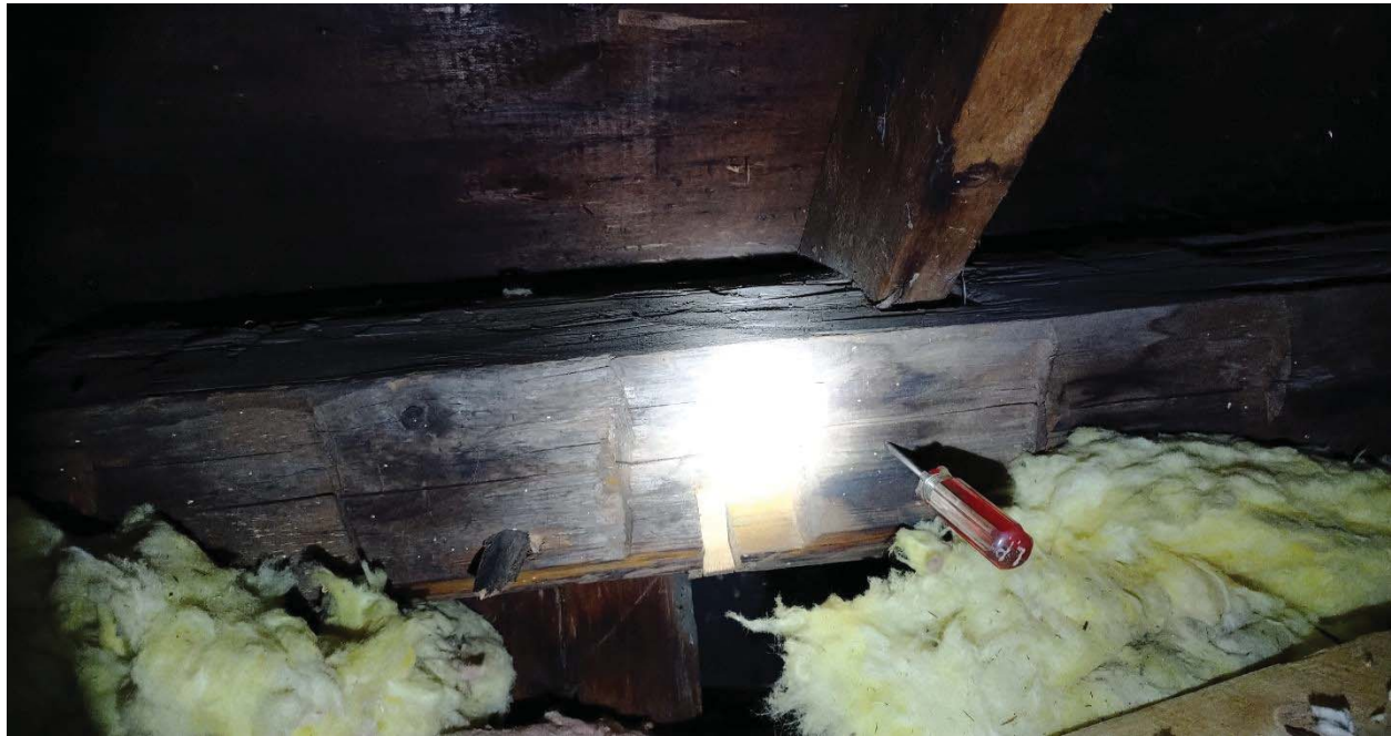
Photo 19: Eave beam has loss of strength due to rot.
