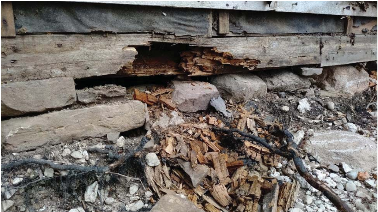
Photo 22: Rot of the perimeter sill beams.
