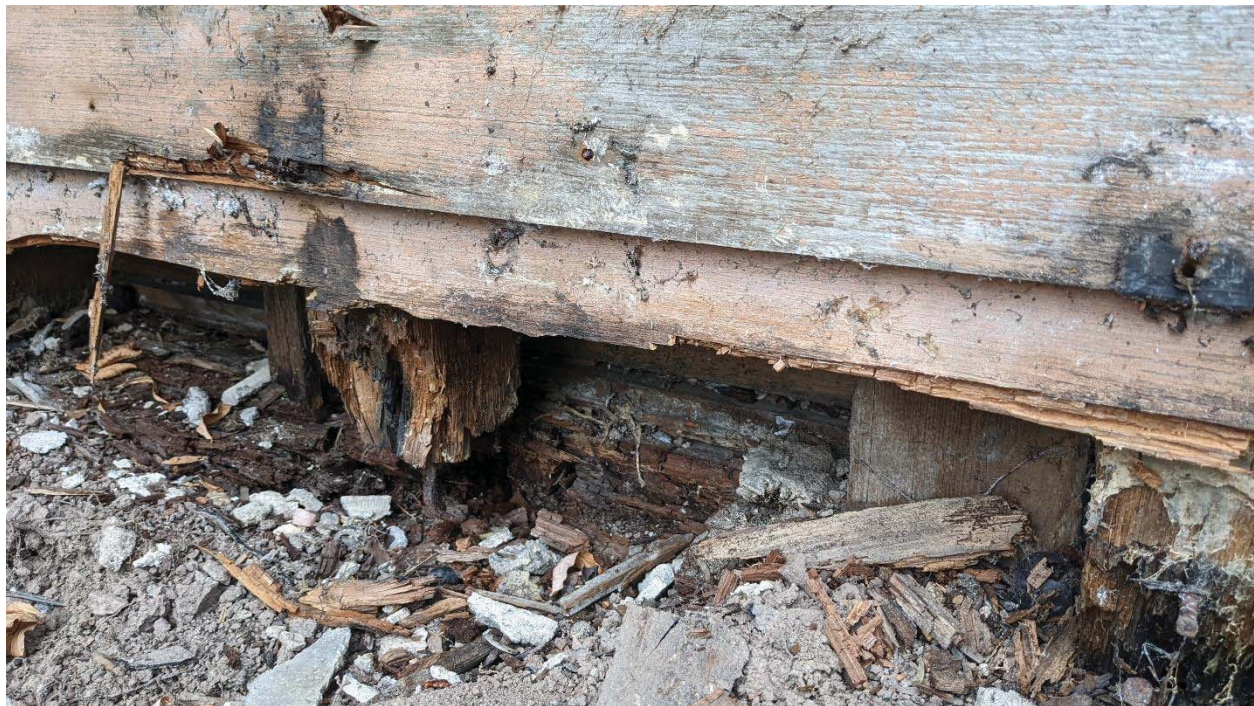
Photo 20: Rot of the exterior studs.
