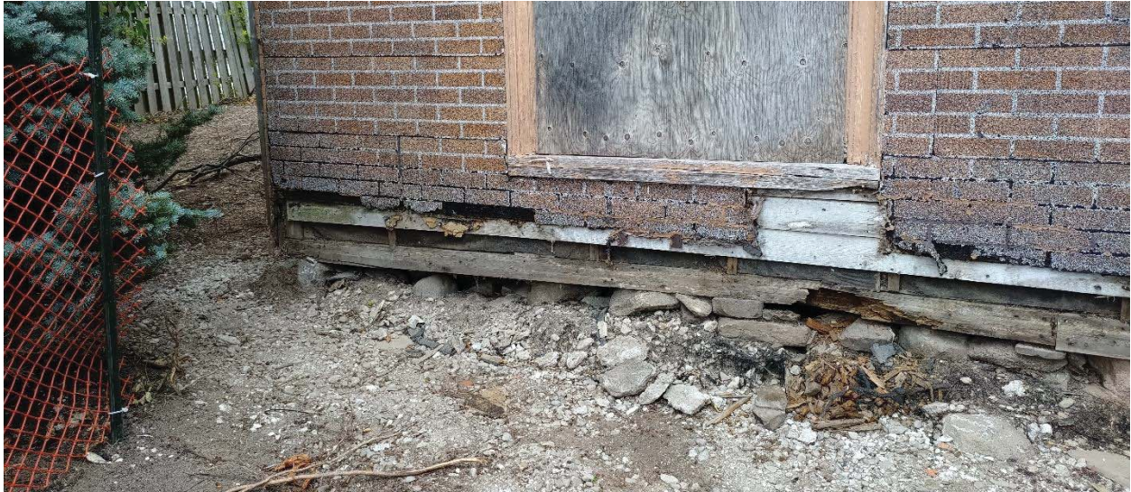
Photo 9: Wood sill on field stone.
