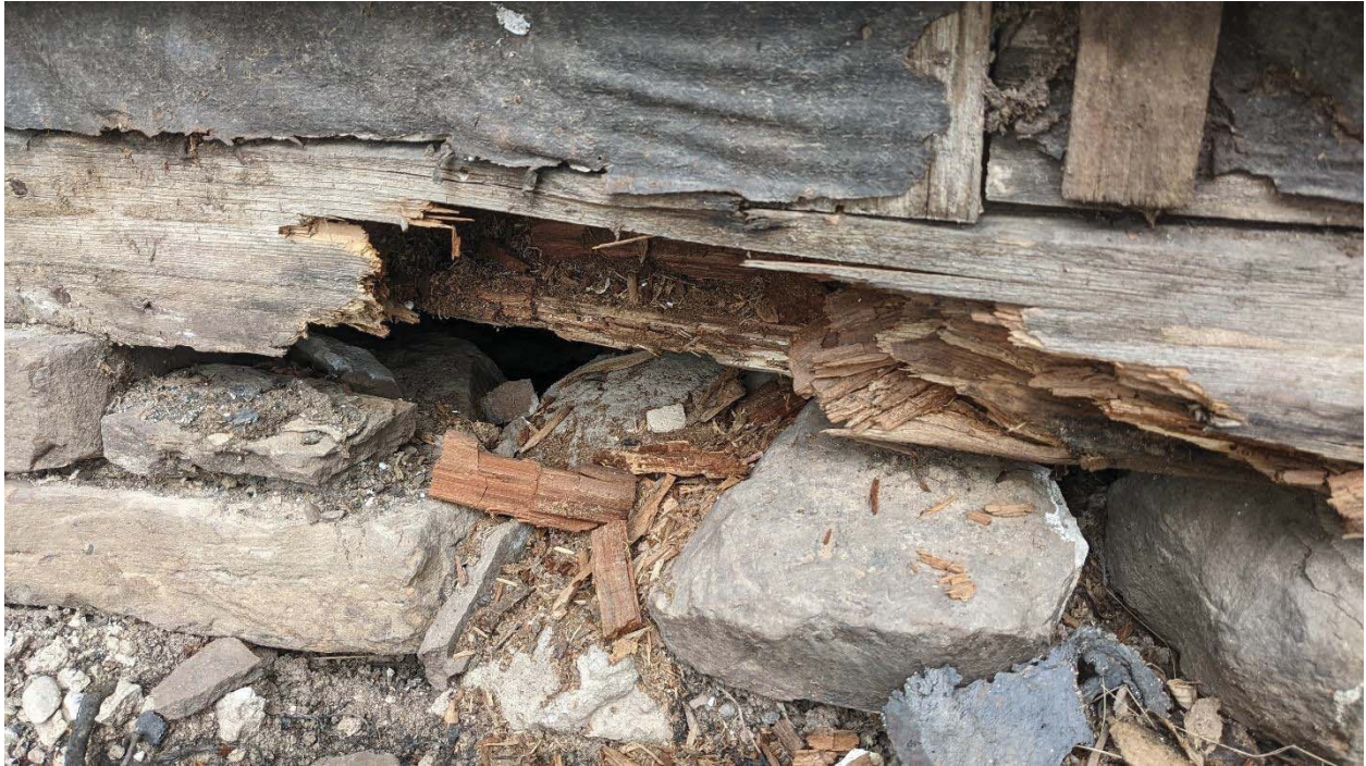
Photo 21: Rot of the perimeter sill beams.
