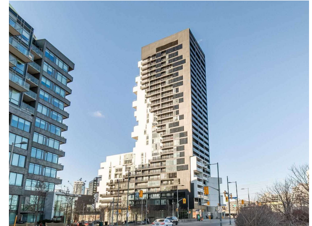
River City Phase 3, Toronto: The signature tower defines the northern gateway
