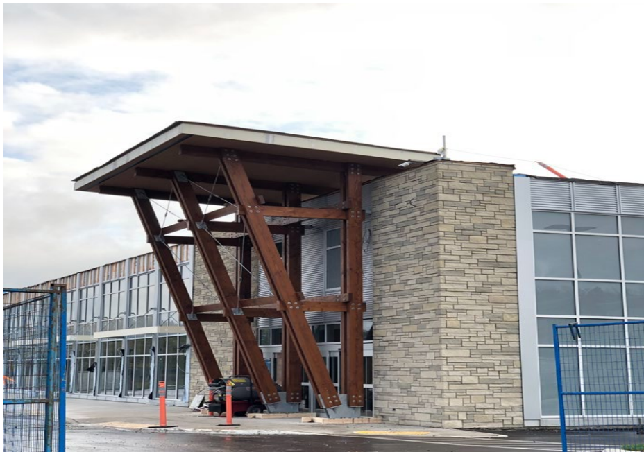
Figure 4 – Example of Proposed structure to support the fascia sign (side view)
